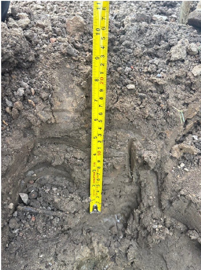
Inspection Pit excavated by client in Plot 133 showing 270mm of topsoil(client-provided photograph)
