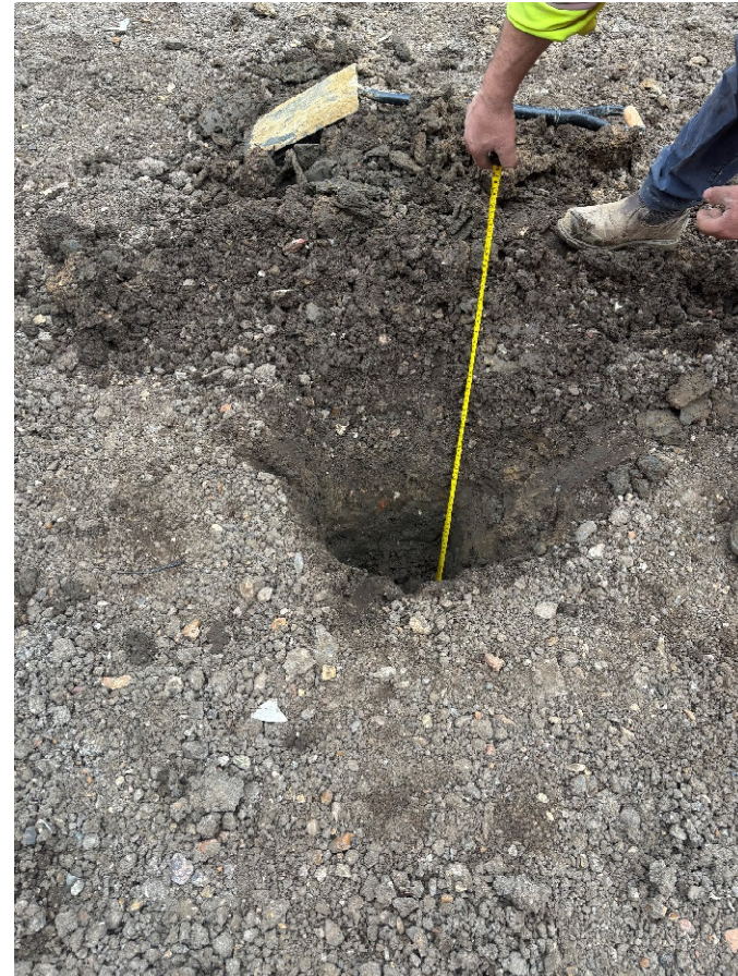
Inspection Pit excavated by client in Plot 141 (client-provided photograph)
