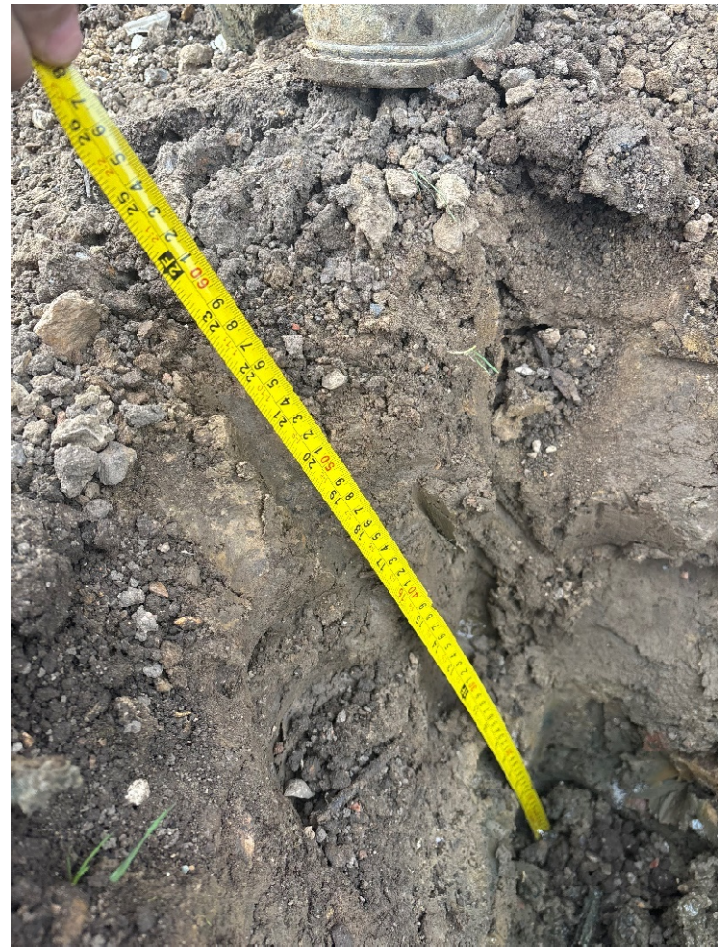
Inspection Pit excavated by client in Plot 142 showing 600mm of clean cover (client-provided photograph)
