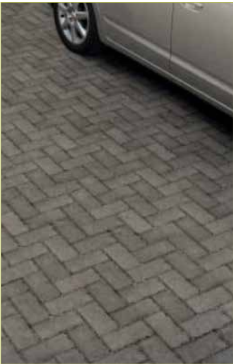
Parking Bays Permeable blocks
