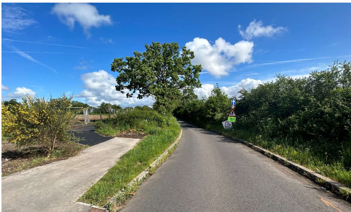
1. View taken on 15 May 2024 looking north up Hyde End Lane with the hedgerow H59 in the foreground. Note the new tarmac pedestrian path which has been recently installed on the western side of the lane.
