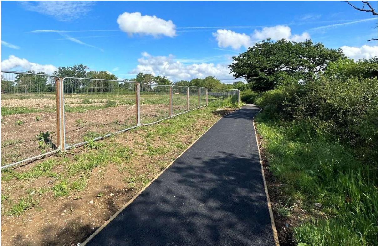
3. View taken on 15 May 2024 looking north up the new tarmac pedestrian path with the development site on the left hand side circa 5m away.
