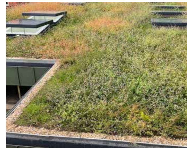
Ecological Enhancements - Extensive Green Roof
