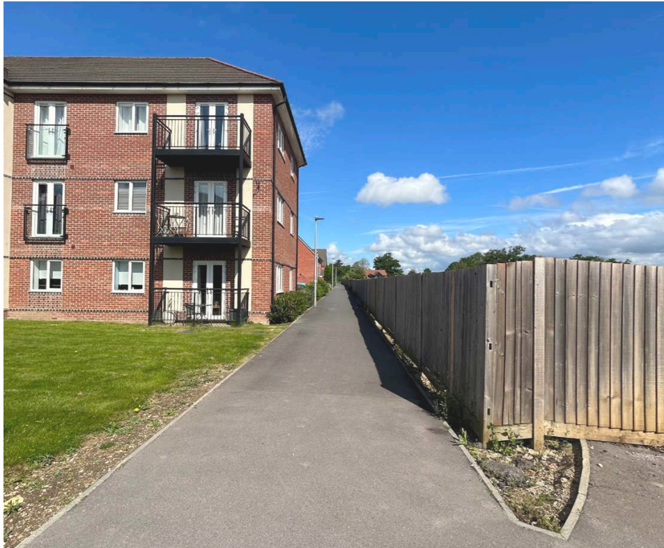
View of pedestrian pathway along the western boundary of the site
