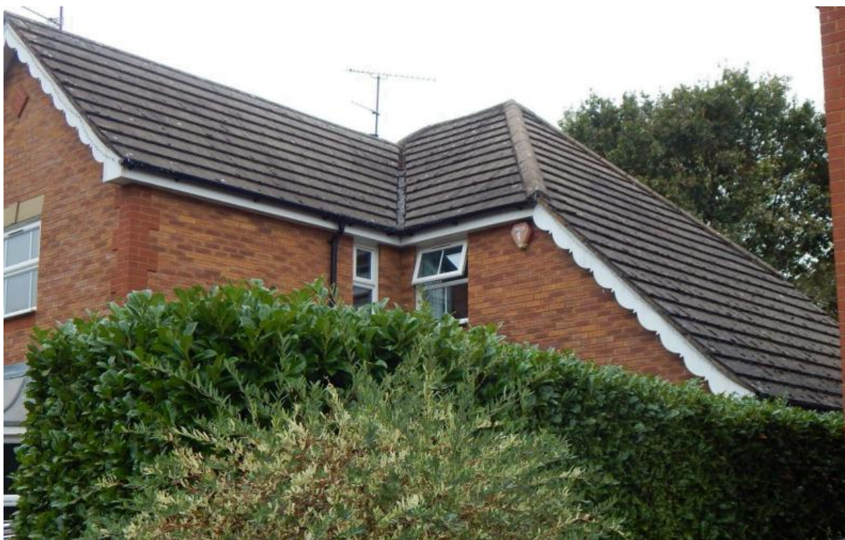
Image 3 – West facing elevation of the property
