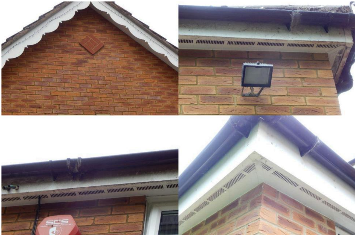
Image 7 – Close view of eaves coverings to demonstrate example of condition throughout
