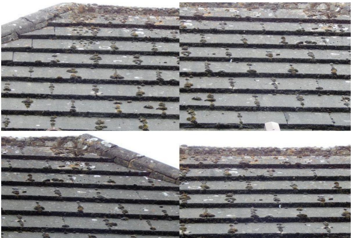
Image 6 – Close view of main tiled roof coverings to demonstrate condition throughout
