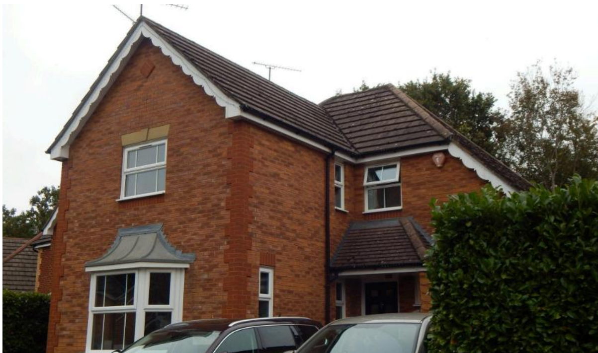
Image 1 – North facing elevation of the property
