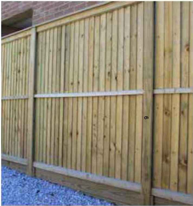
Typical Fence View
