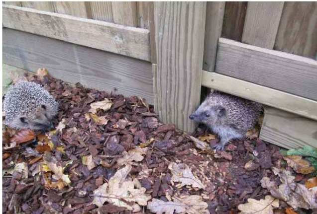
Typical hole on the gravel board (base of fence)
