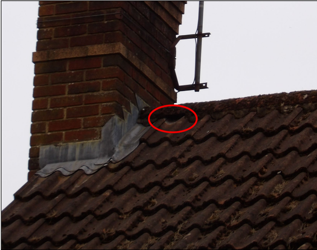
Figure 5. Missing mortar from ridge. Wychwood House, Finchampstead. 20.05.25
