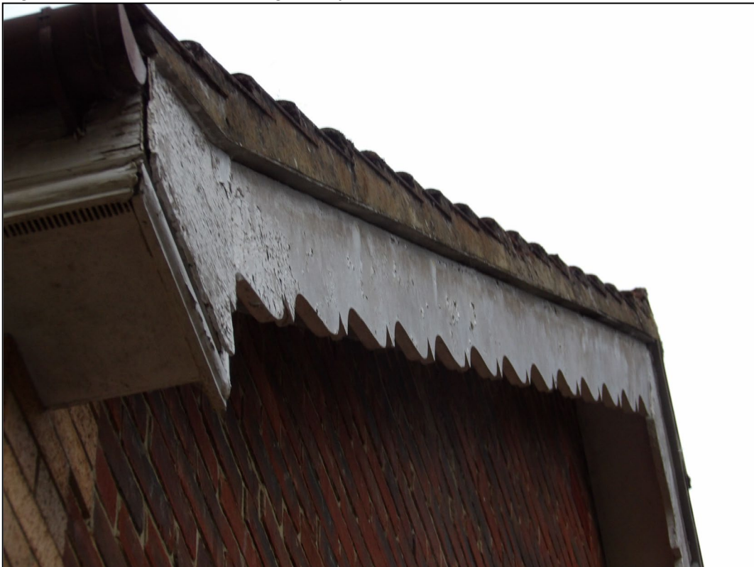
Figure 6. Example sealed verges. Wychwood House, Finchampstead. 20.05.25
