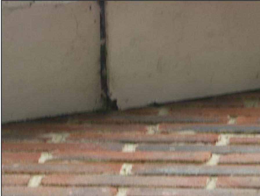
Figure 7. Gaps with soffit and mortar on property. Wychwood House, Finchampstead. 20.05.25
