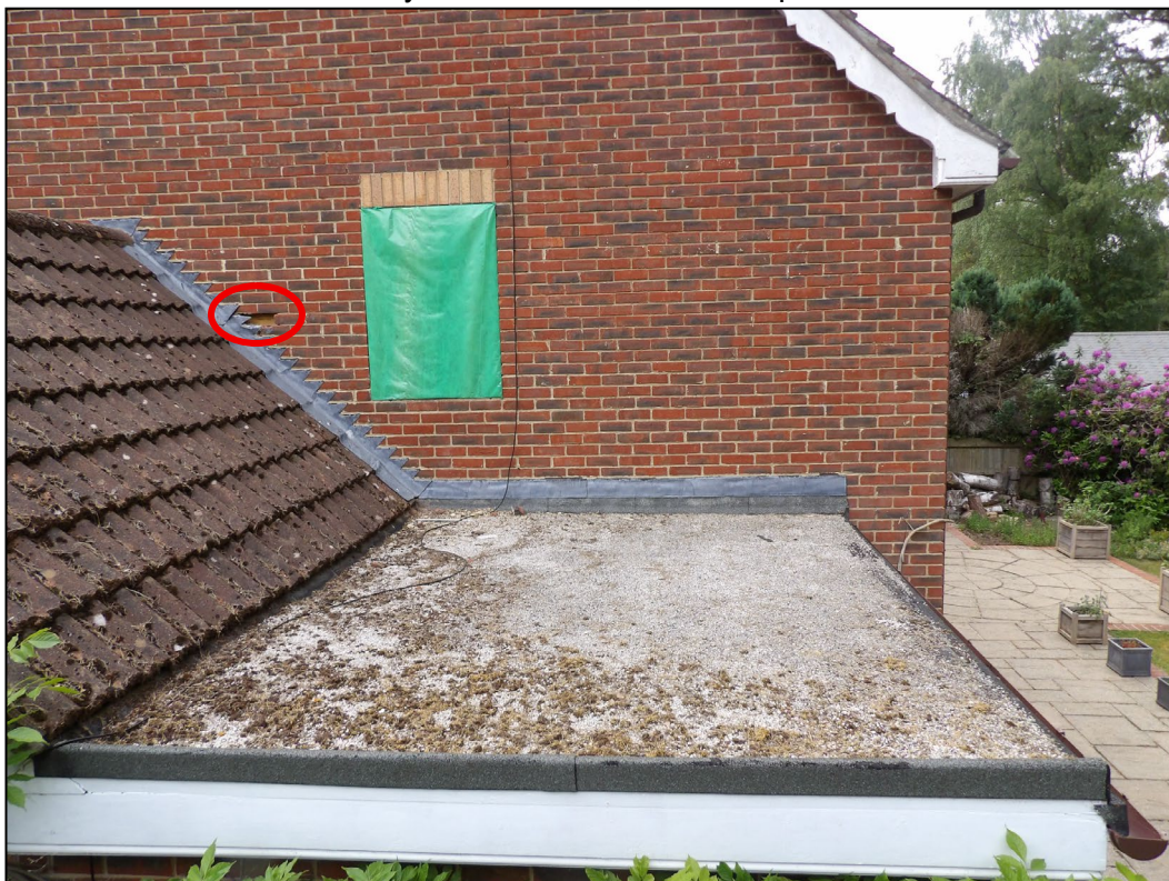
Figure 9. Temporary sealing of removed window and gap where the missing brick was and rear flat roof section. Wychwood House, Finchampstead. 20.05.25
