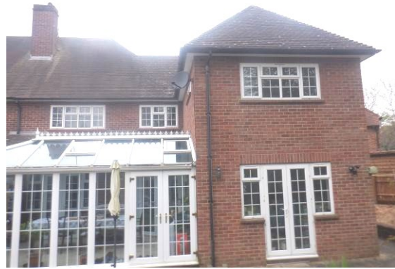
Photograph 2. Rear and side of property viewed from the southeast.
