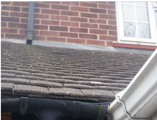
Photograph 3. Tight clay roof tiles (rear elevation).
