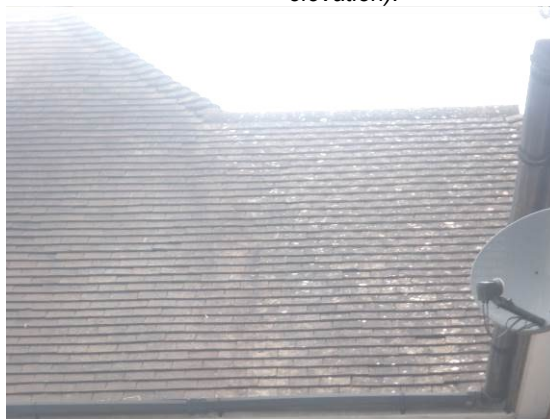
Photograph 5. Intact ridge and hip tiles and mortar (rear elevation).
