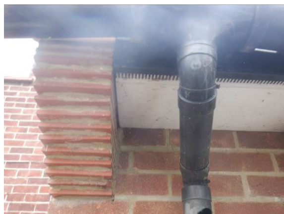
Photograph 11. Intact soffit tight to brickwork (rear elevation).
