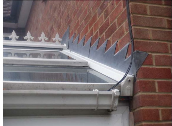
Photograph 7. Lead flashing sealed along the conservatory roof (rear elevation).
