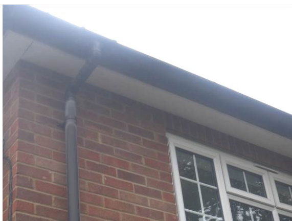
Photograph 10. Intact soffit tight to brickwork (side elevation).
