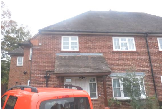
Photograph 1. Front of property viewed from the northeast.
