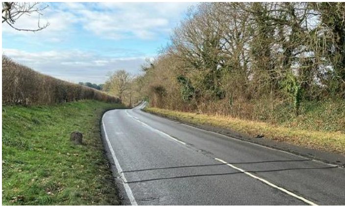
Photograph 3: Eastbound ATC Location
