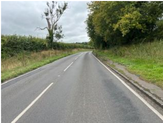
Figure 1: Visibility to the rear of stationary traffic.
