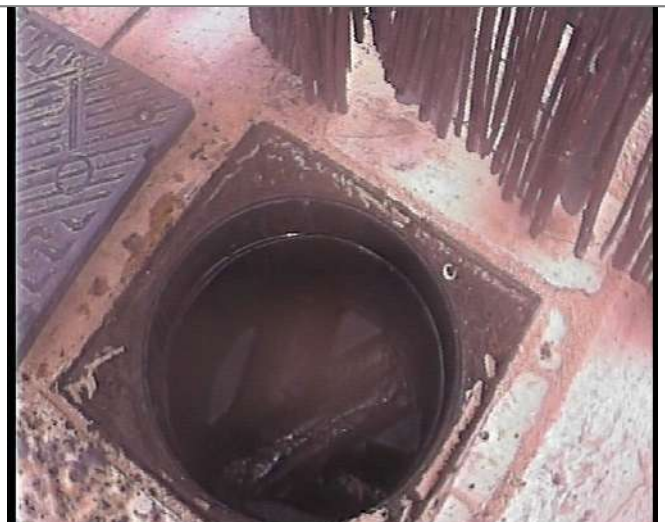
Manhole / Access Point: FWMH2 Internal
