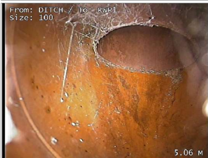
Finish node type, rodding eye, reference number RWP1
