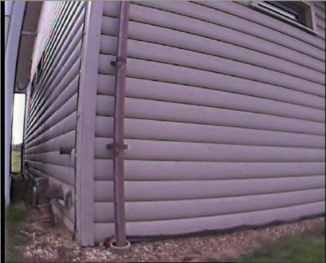
Manhole / Access Point: RWP1 Location
