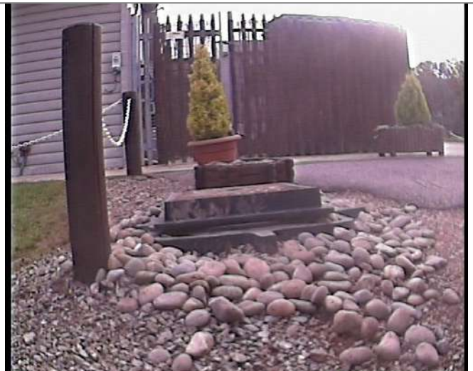
Manhole / Access Point: PUMP CHAMBER Location
