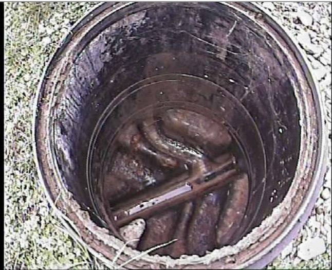
Manhole / Access Point: FWMH1 Internal
