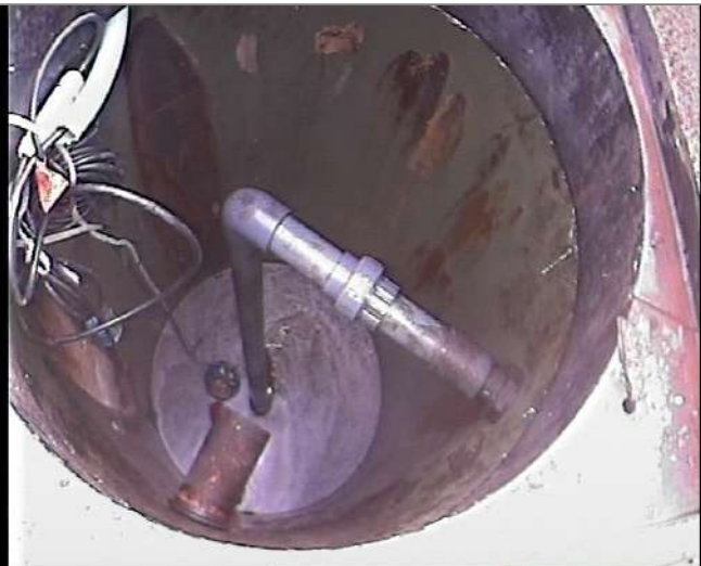
Manhole / Access Point: PUMP CHAMBER Internal
