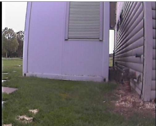
Manhole / Access Point: LAT1 Location
