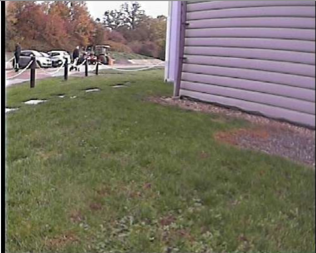
Access problems: BURIED FOUL M/H ON THE CORNER OF THE BUILDING
