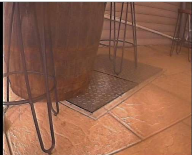
Manhole / Access Point: GREASE TRAP Location
