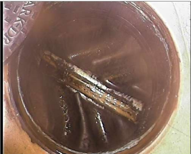
Manhole / Access Point: FWMH3 Internal
