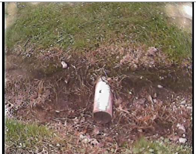
Manhole / Access Point: DITCH Location
