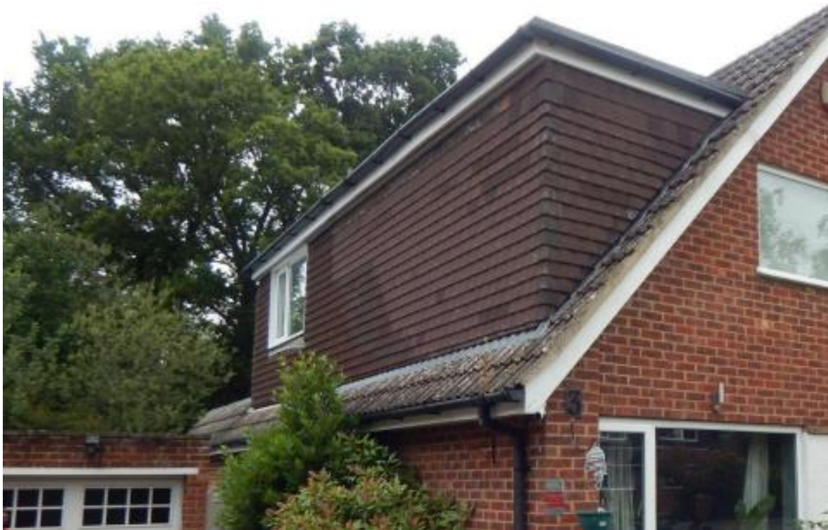
Image 5 – West facing elevation of the property
