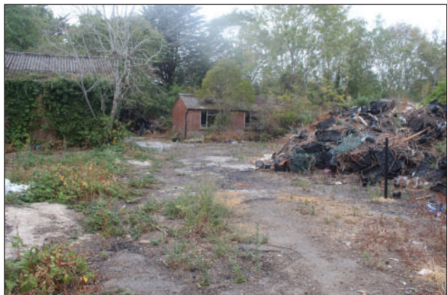
Plate 4. View of site, looking north-west.
