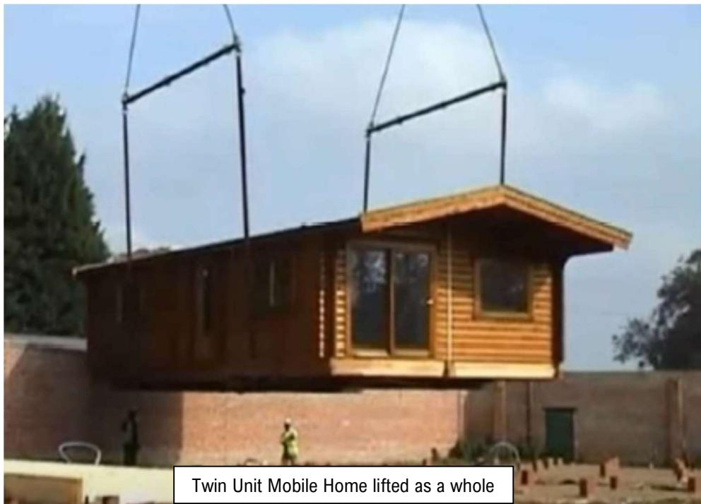
Due to the size of the proposed twin unit caravan, the road and site access complexities, the independently assembled sections will be wheeled into position with the connection being the final act.
