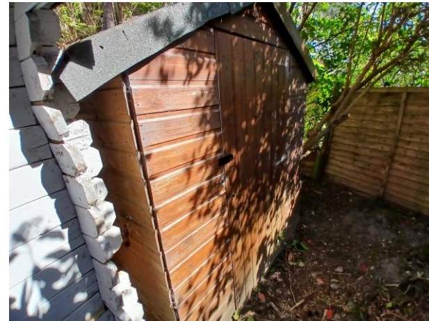
The southern elevation of B3.
