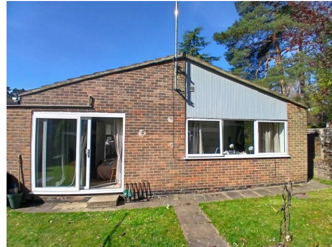
Eastern elevation of B1.
