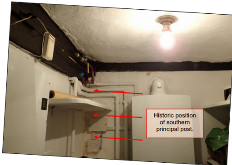
Figure 36. South-west corner of the Utility Room.
