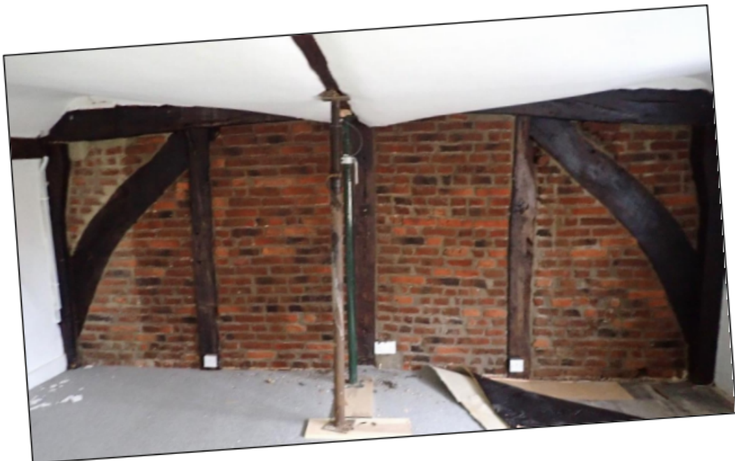
Figure 37. General view of the west wall on the 1 st floor.
