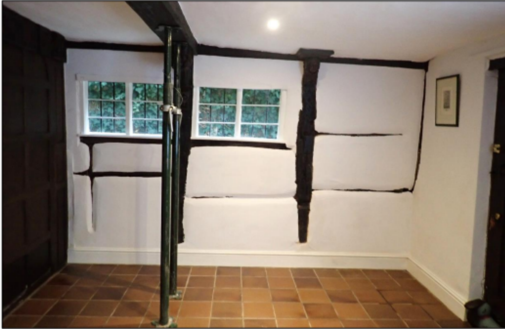
Figure 28. General view of the west wall from the Dining Room.
