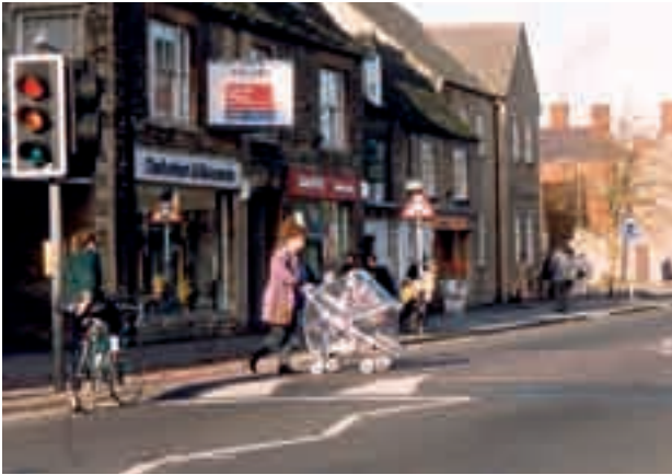
Fig. 2.6 Humped pelican and zebra crossings
