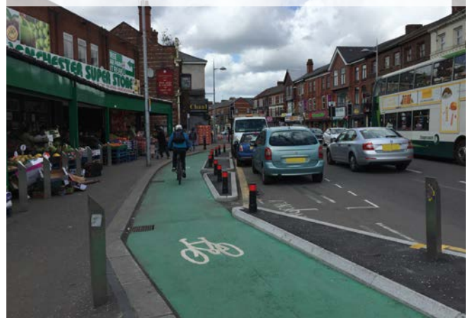
Figure 1.10: Example of kerb-segregated cycle track
