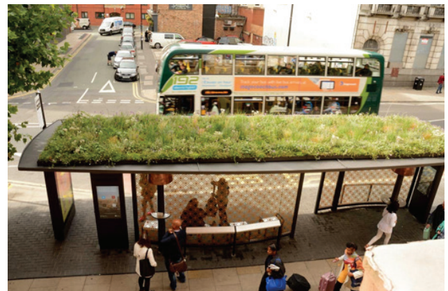
Figure 37: 'Concept shelter' with screen in centre of footway arranged to provide shelter on either side. Note also the green roof. (Photo courtesy of Transport for Greater Manchester)
