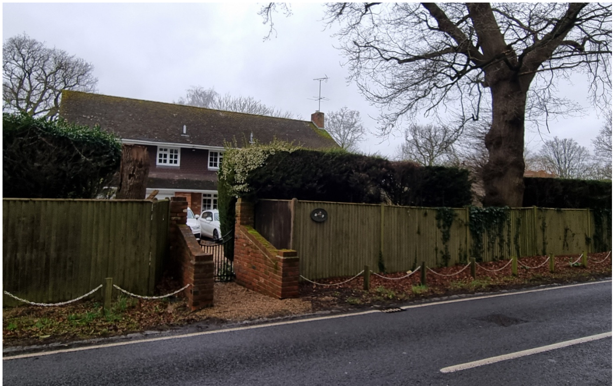
Pedestrian gate and walls to be removed to form new vehicular exit onto Wokingham Road. No dropped kerb is required as the road surface is flush with the ground along this side of the road.
