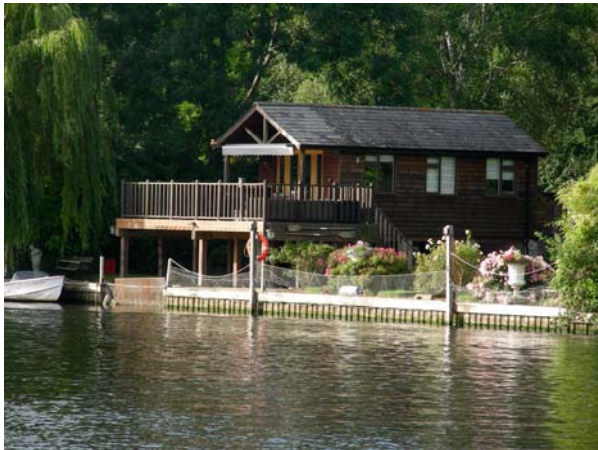
view from the south
