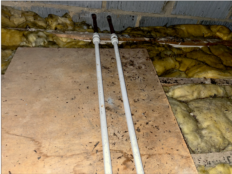
Photograph 4: Showing the scattering of brown long-eared bat droppings recorded within the attic space above the single-storey extension, which will remain unaffected by the works.
