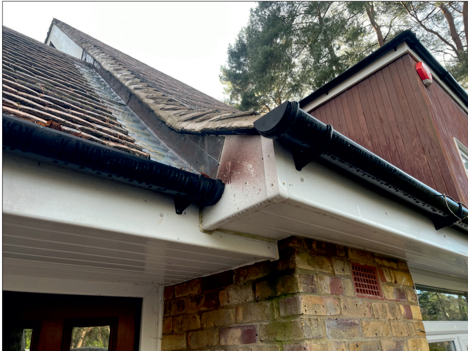
Photograph 2: Showing the well-sealed roof tiles and soffits/fascias.
