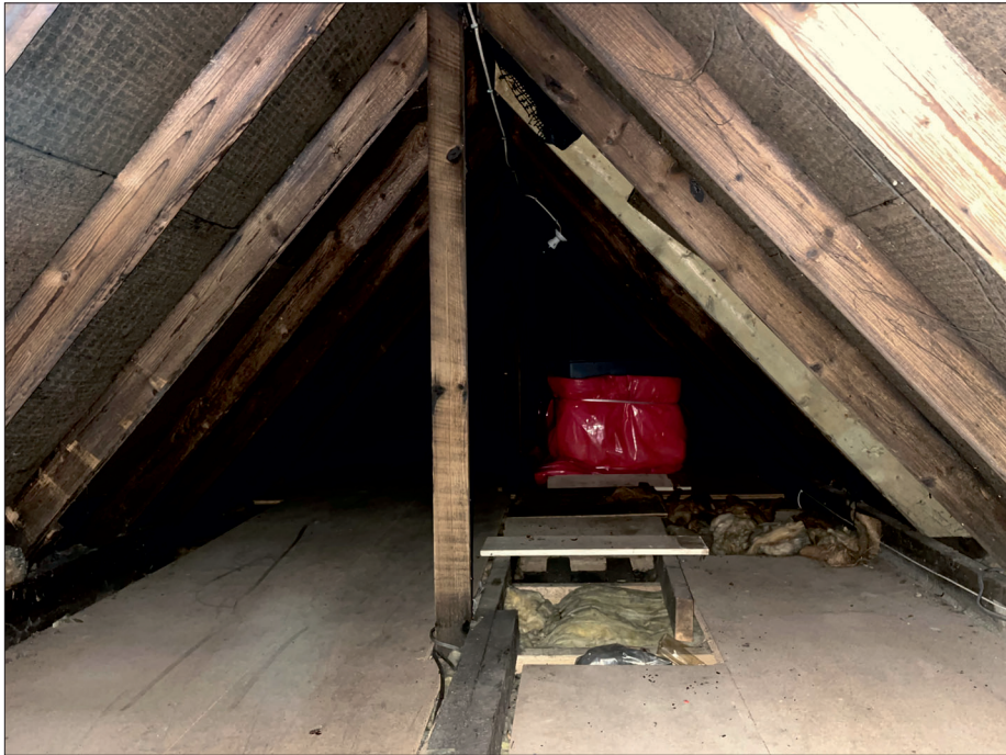
Photograph 3: Showing the main attic space within the property, which will remain unaffected by the works.
