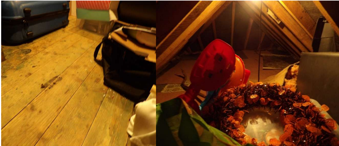
Figure 3. Bitumen felt in good condition.
