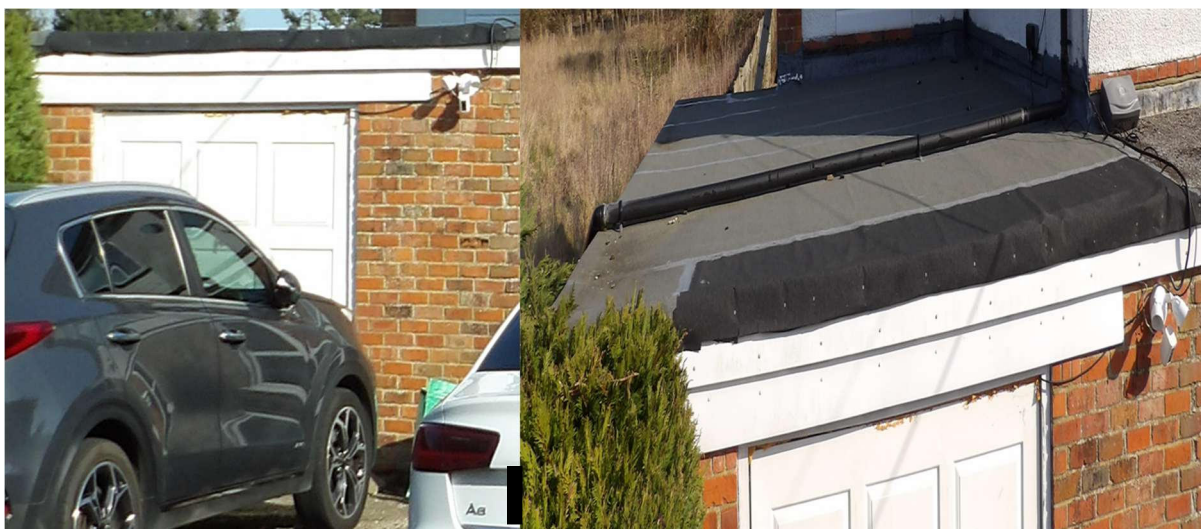
Figure 14. Garage soffits and fascias.
