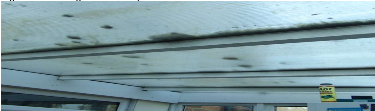
Figure 5/6. OSB lining garage flat roof.
