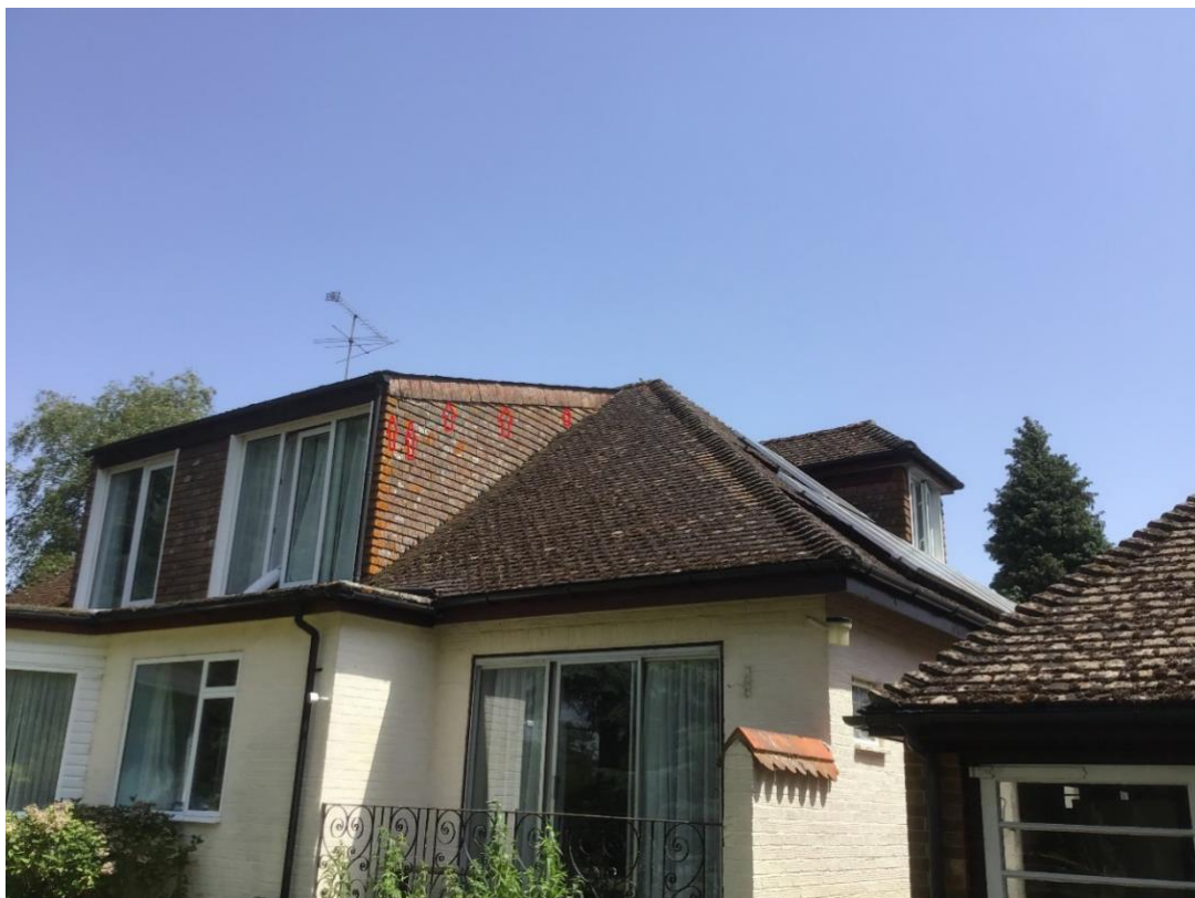
Figure 2. Northern and western elevations looking north-east. Red arrows indicate potential access points into under-tile spaces.
