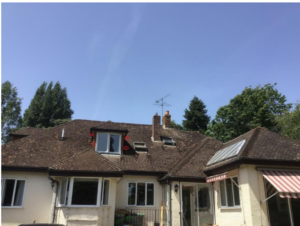
Figure 4. Southern elevations looking north-west. Red arrows indicate potential access points into under-tile spaces.
