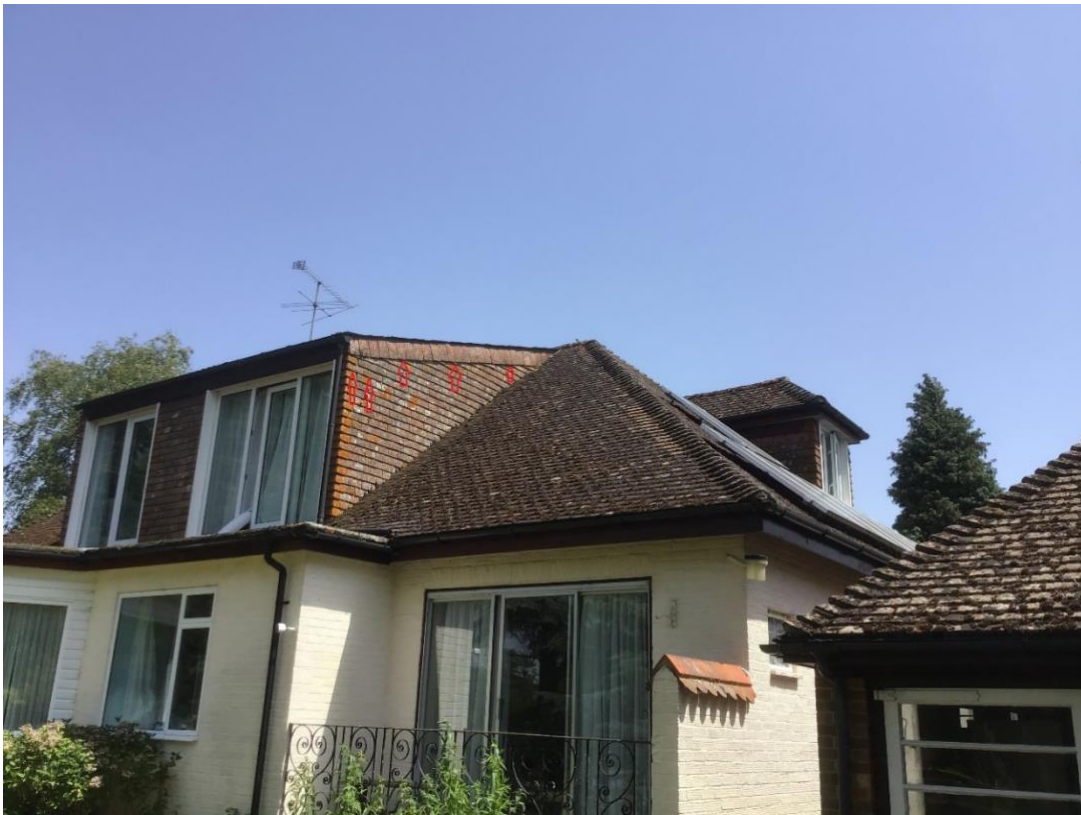
Figure 3. Northern and western elevations looking north-east. Red arrows indicate potential access points into under-tile spaces.
