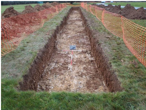
Plate 15 South facing shot of Trench 4
