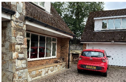
Figure 6- current set back living room wall
