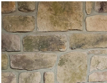
Figure 18- Stone to be weathered Cotswold blend stone slips.
