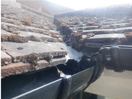
Photograph 6. Tight led flashing on the hip roof of the rear extension.
