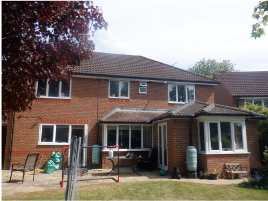
Photograph 1. Rear of the house viewed from west.
