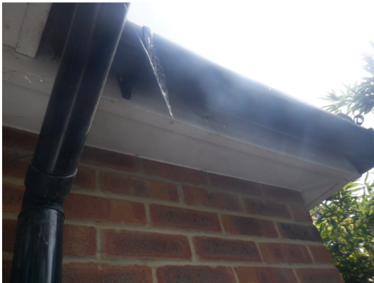
Photograph 8. Intact soffits tight to the brick of the property.
