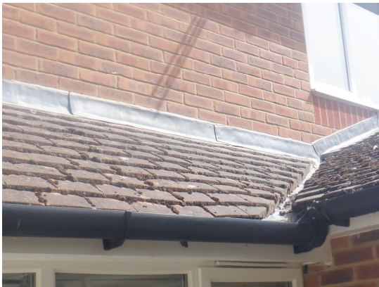
Photograph 2. Intact/tight plain roof tiles on the rear elevation.
