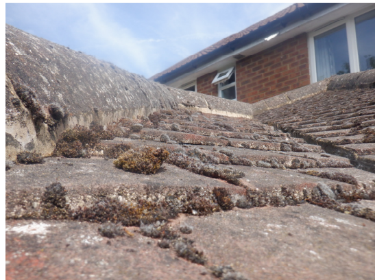
Photograph 3. Intact mortar between hip tiles and plain roof tiles on the rear extension.
