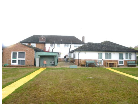
2. Rear of property viewed from north.
