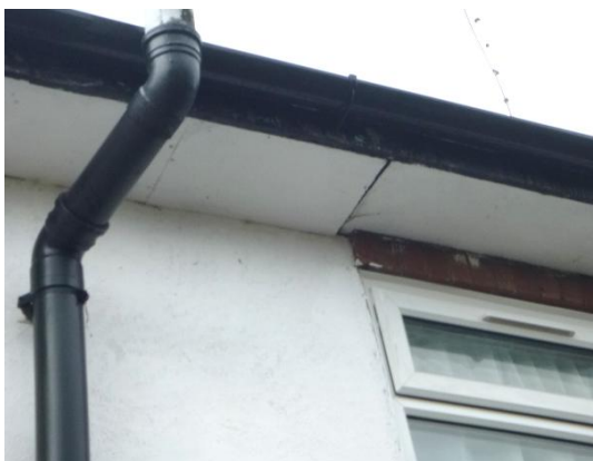
7. Separating soffit boards (rear elevation).
