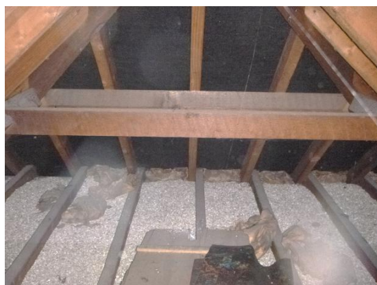
19. Eaves filled with fibreglass and paper.
