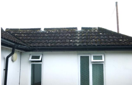
10. Concealed flat roof on single-storey extension (rear elevation).
