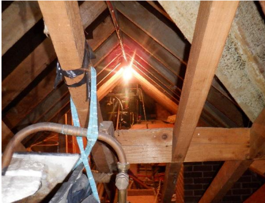
14. Roof void viewed from eastern end.
