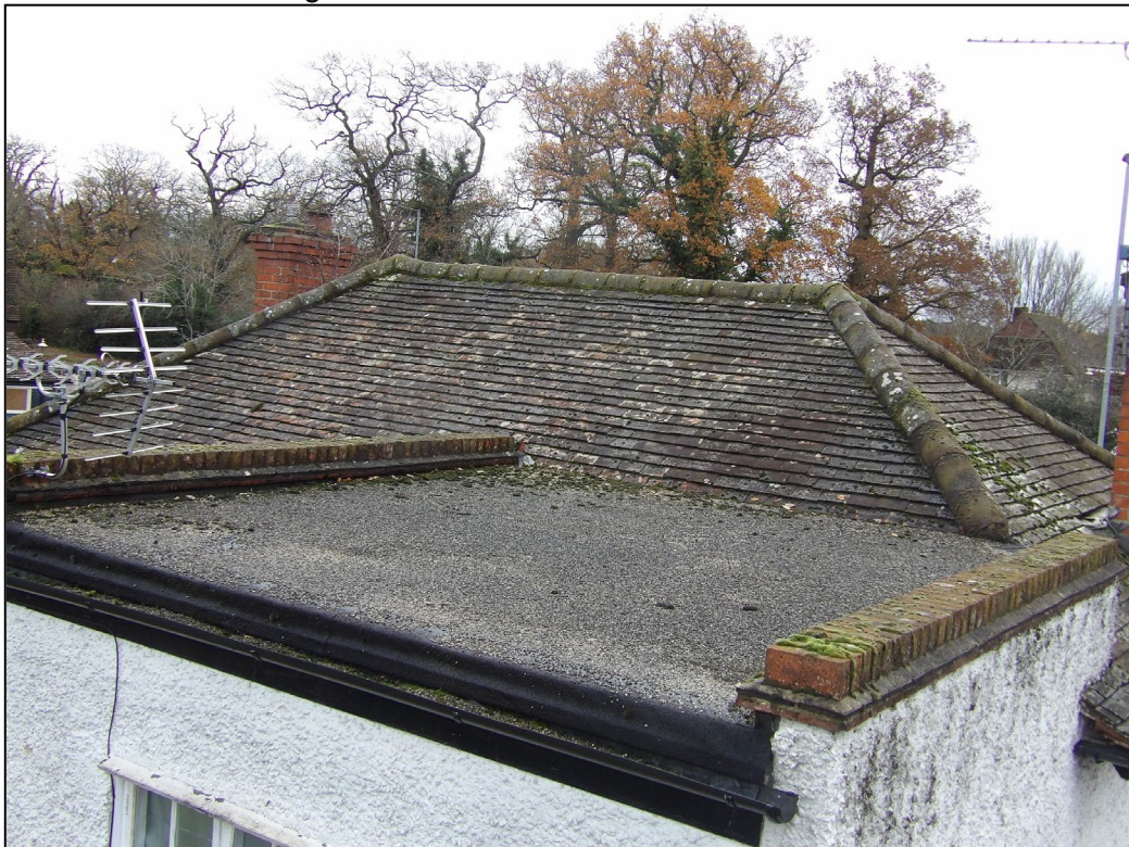
Figure 6. Example sealed bitumen felt on rear, two-storey flat roof extension. 220 London Road, Wokingham. 09.12.25
