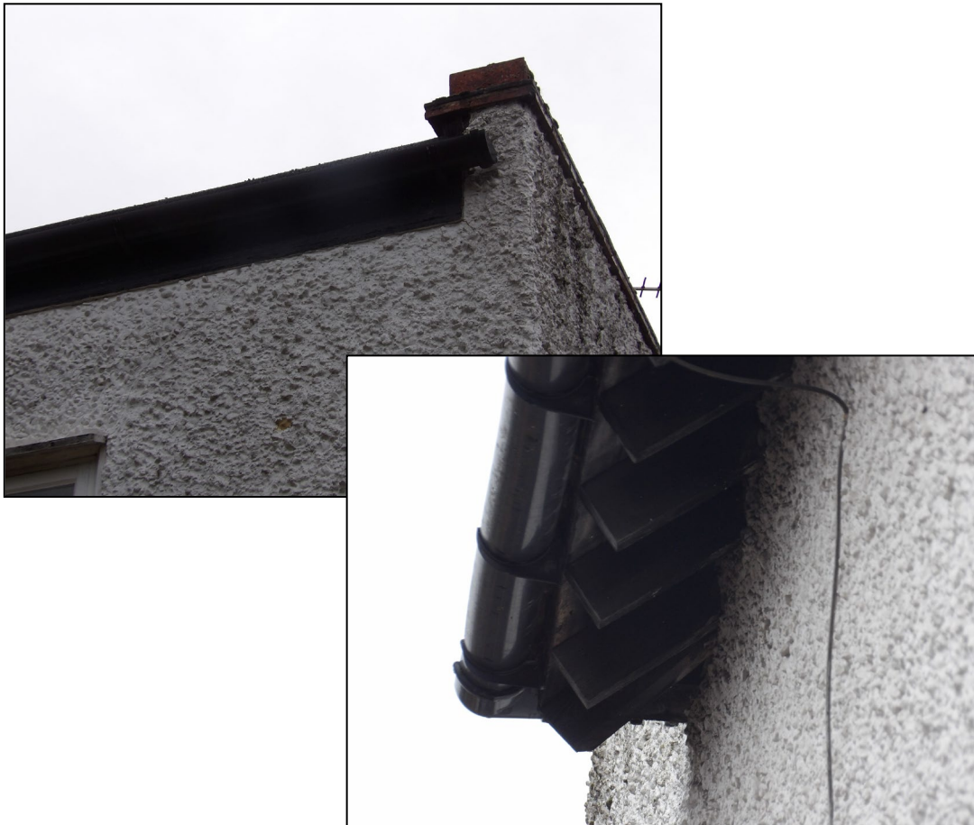
Figure 8. Example sealed fascias and eaves. 220 London Road, Wokingham. 09.12.25
