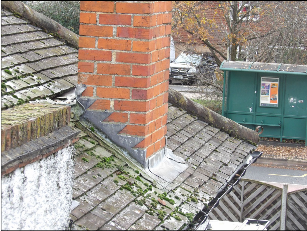
Figure 5. Example sealed lead flashing. 220 London Road, Wokingham. 09.12.25
