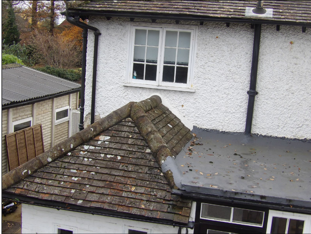
Figure 8. Example sealed fascias and eaves. 220 London Road, Wokingham. 09.12.25
