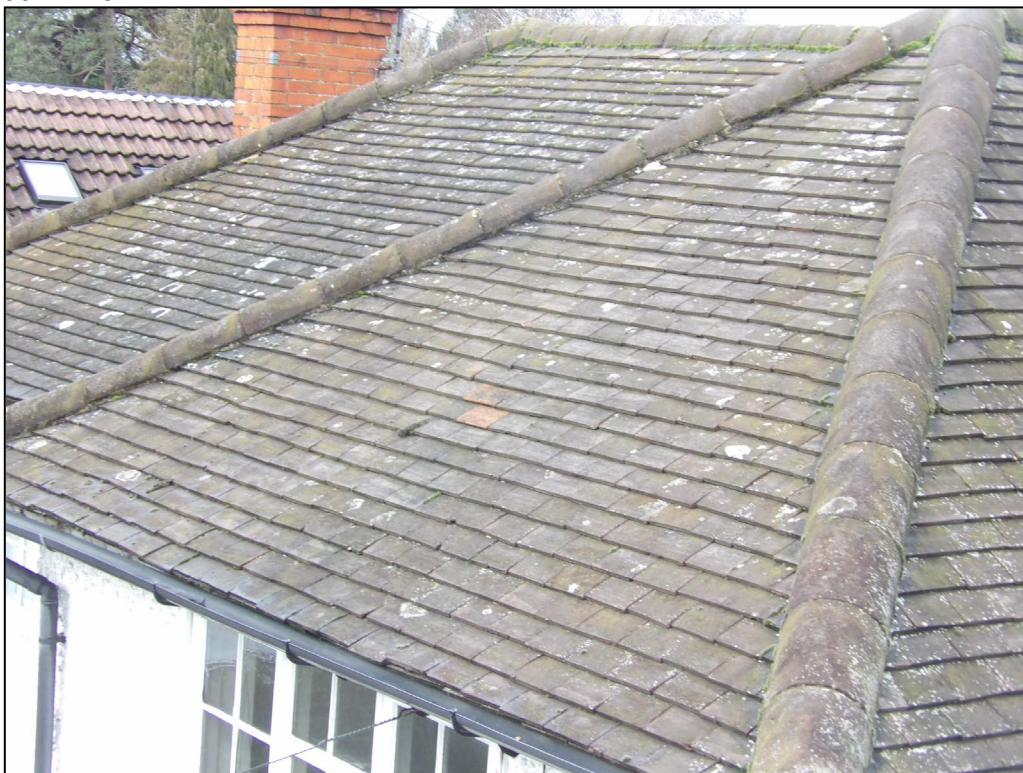
Figure 4. Example well fitted roof, ridge and hip tiles. 220 London Road, Wokingham. 09.12.25
