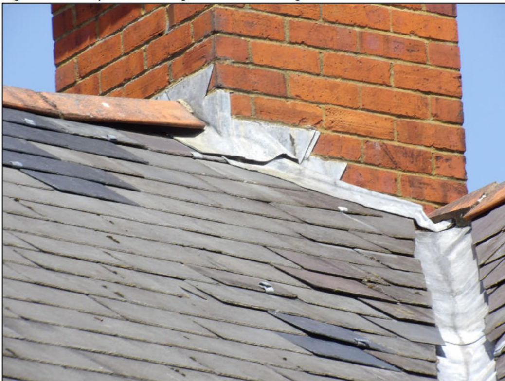
Figure 6. Example raised ridge tile/lead flashing. Lea Heath House, Hurst. 23.06.26
