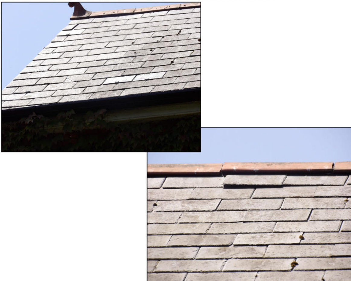
Figure 5. Example raised roof tiles. Lea Heath House, Hurst. 23.06.26
