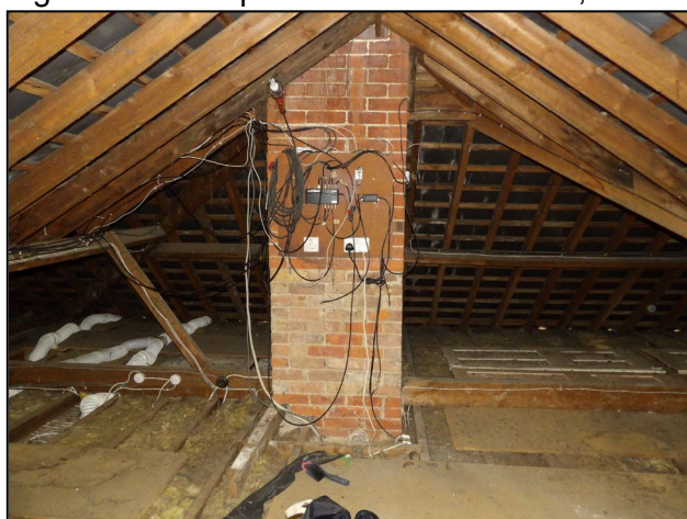
Figure 11. Loft space. Lea Heath House, Hurst. 23.06.26
