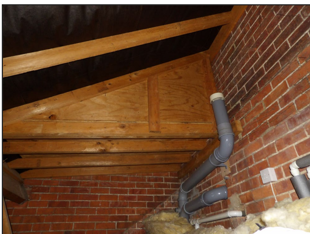
Figure 13. Mono-pitched loft space and membrane lining to tiles. Lea Heath House, Hurst. 23.06.26
