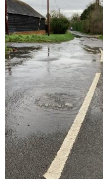
Thames Water pumping station ineffective
