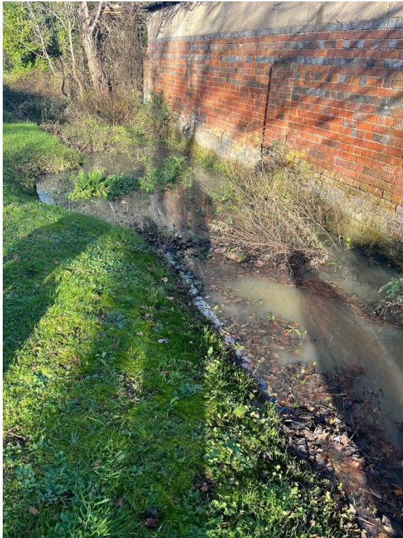
4b. Site visit - ditch downstream from culvert (taken on 28 November 2023)
