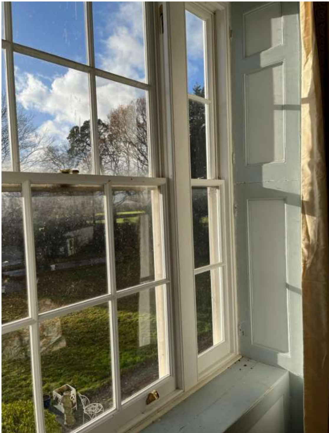
Figure 9. Previously restored window to toom FF4
