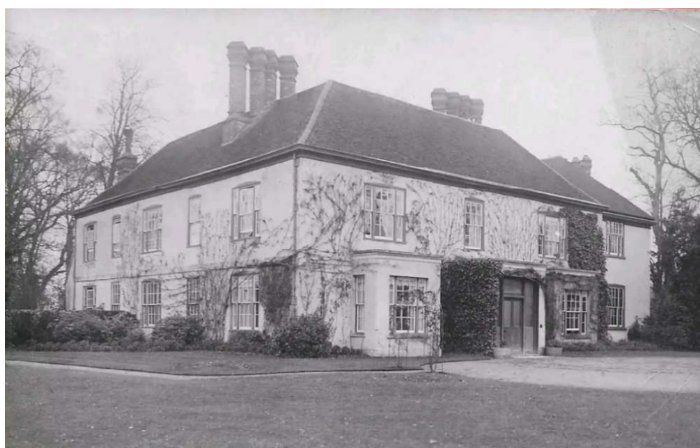
Figure 5. Photograph of the front elevation britishlistedbuildings.co.uk
