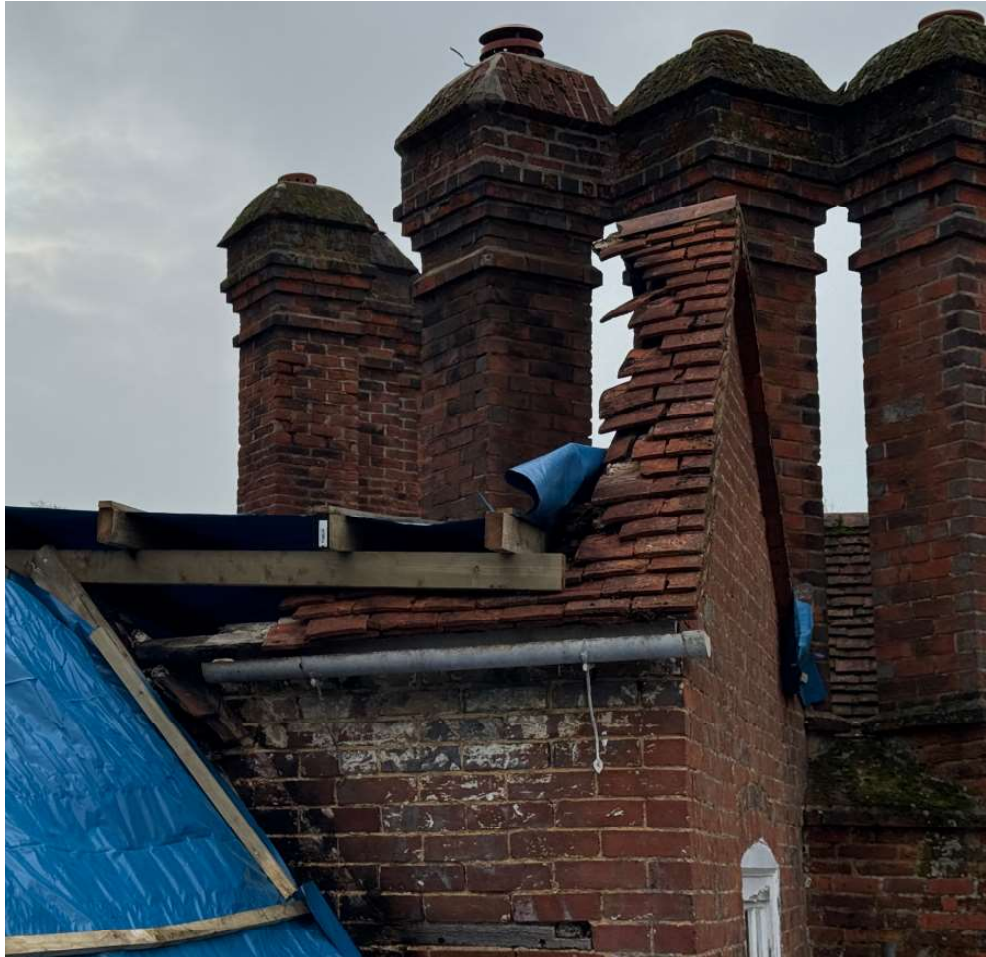
Facing brickwork to gable end of room SF3. The window to the staircase is visible. Note how the flank wall between SF3 and SF2 is a single skin brickwork wall and so exhibits a running bond. This is the gable noted in the structural engineers' report as needing supporting.
