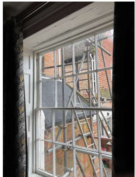
Here is the sash window to room GF5 from the exterior and then interior. The windows that require replacement will use the existing windows as a template. Under a previous application to the property some of the windows were replaced from UPVC back to timber sash windows. The same window supplier would be recommended for this application.
