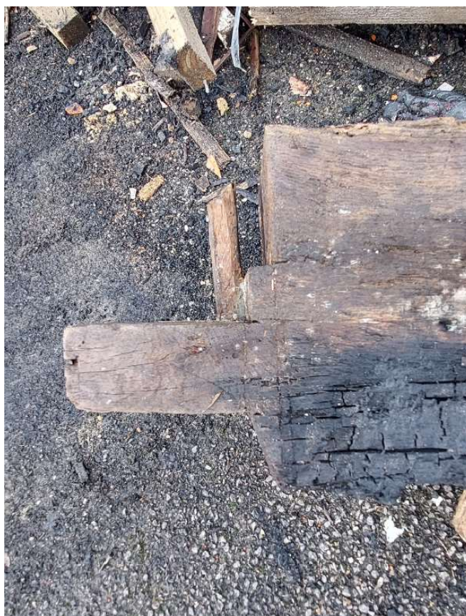
Figure 7. Tenon detail to floor beam
