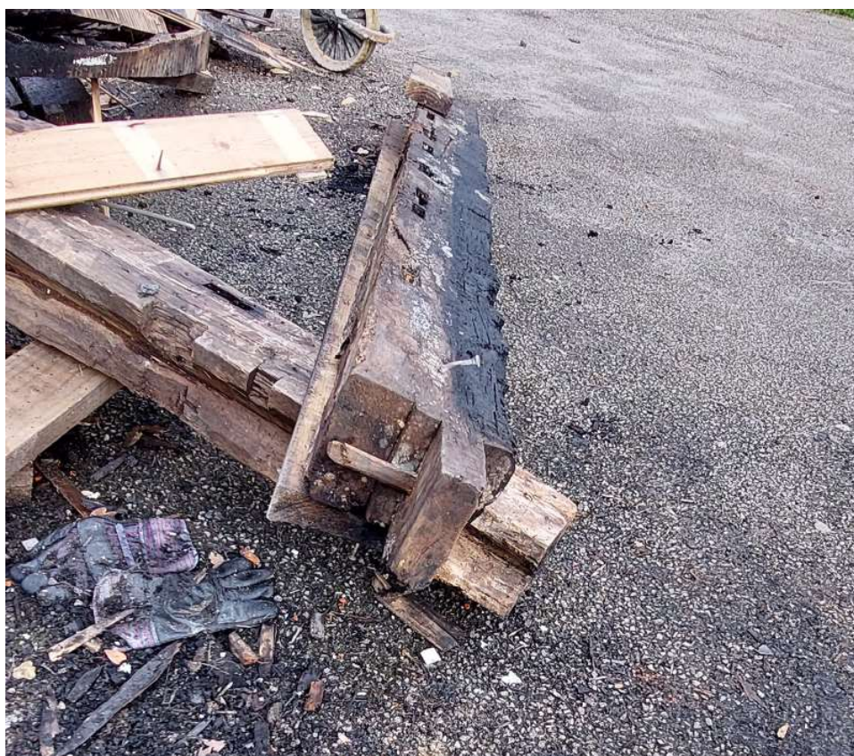
Figure 8. Tenon detail to floor beam
