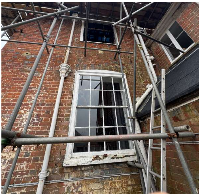
Here is the sash window to room GF5 from the exterior and then interior. The windows that require replacement will use the existing windows as a template. Under a previous application to the property some of the windows were replaced from UPVC back to timber sash windows. The same window supplier would be recommended for this application.
