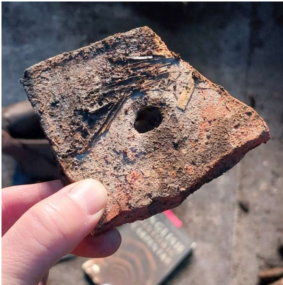
Figure 6. A broken tile from the roof. Evidence of torching can be seen with a mortar and straw mix
