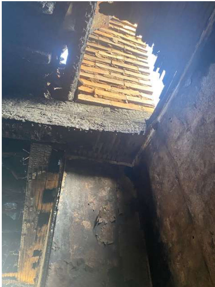
Photograph 9 & 10- Oak beam – corbel chimney stack
