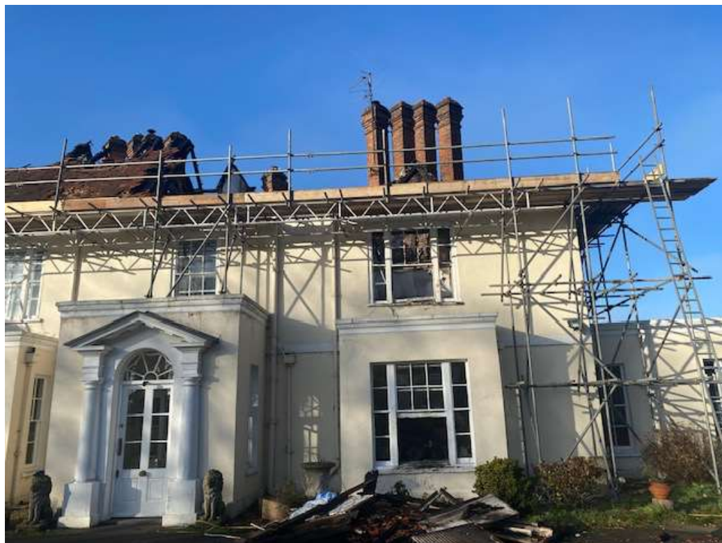
Photograph 1 & 2 -Front elevation (East Facing)
