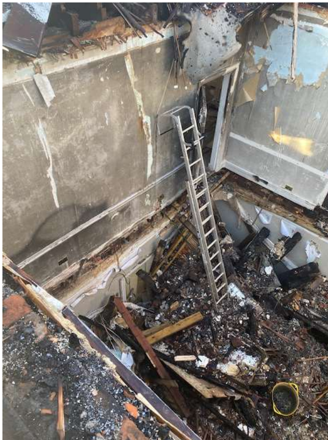
External walls and point of fire damage
