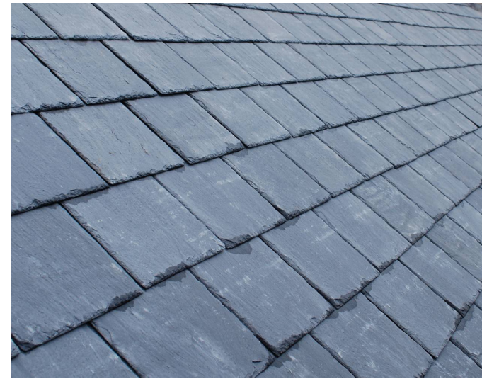
Roof - Natural Slate
