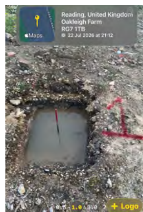
Pit - 1 drained; third attempt.
