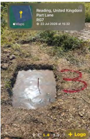
Pit 3 - filled second attempt.
