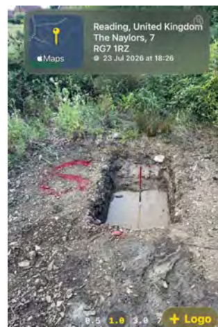
Pit - 6 drained; third attempt.
