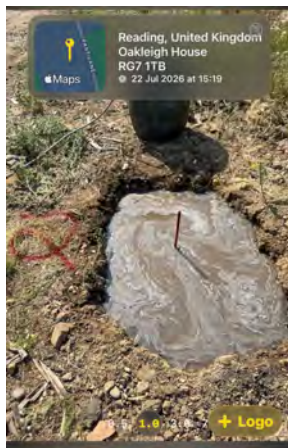
Pit 2 - filled second attempt.
