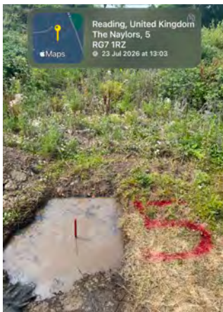
Pit 5 - filled third attempt.
