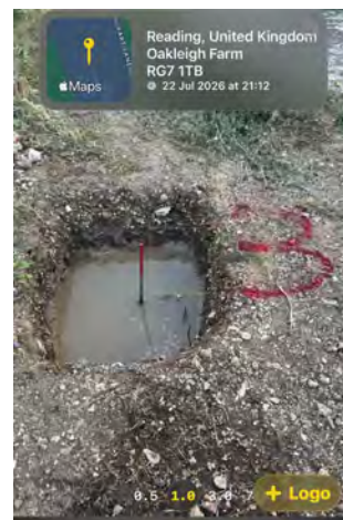
Pit - 3 drained; third attempt.
