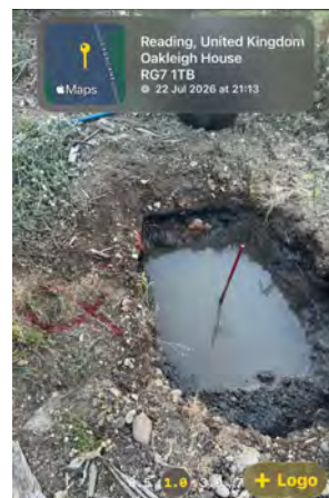
Pit - 2 drained; third attempt.
