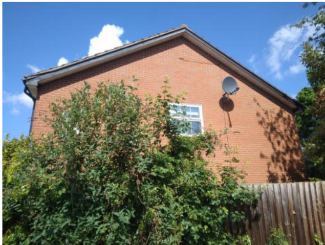
Building B1 – Eastern elevation
