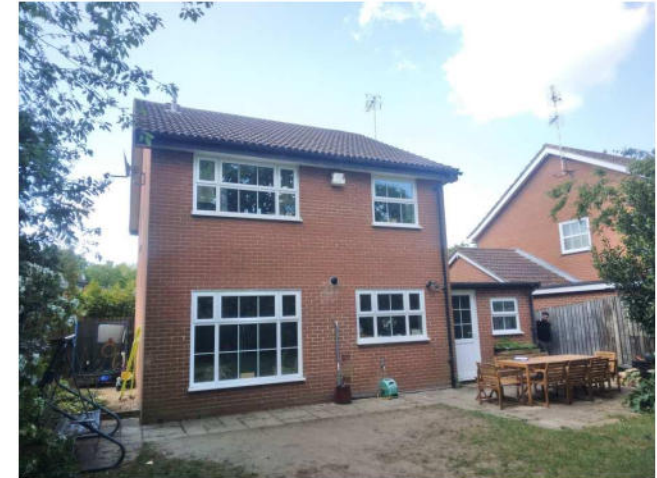
Building B1 - Northern elevation
