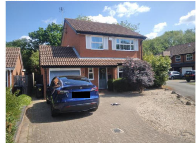
Building B1 – Southern and western elevations
