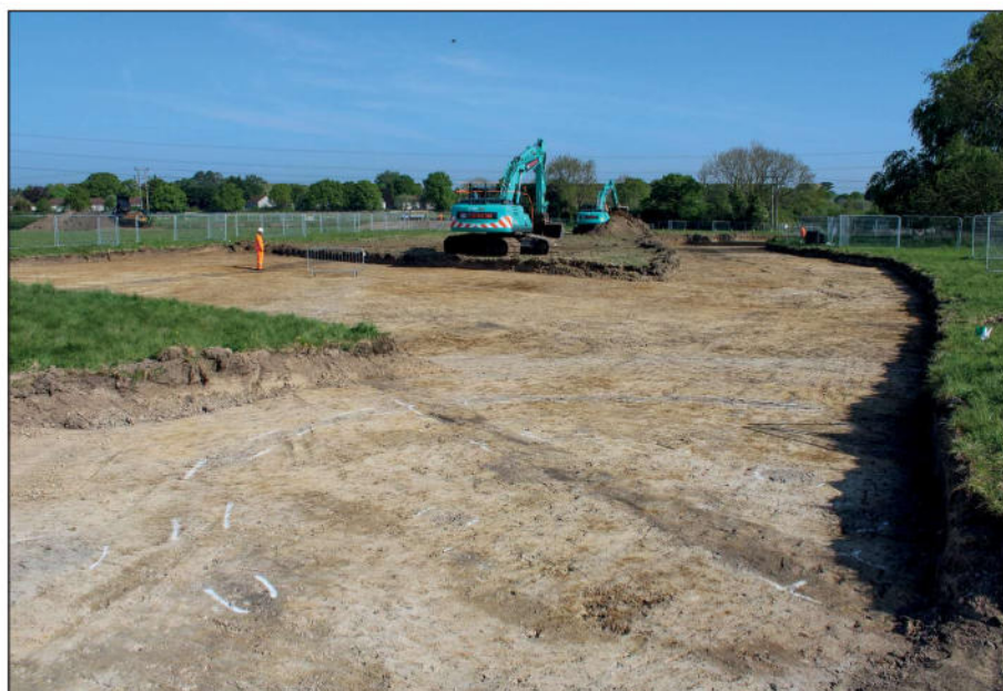
Figure 11. Ditch 10207 cut by ditch 10202, viewed from the south-east
