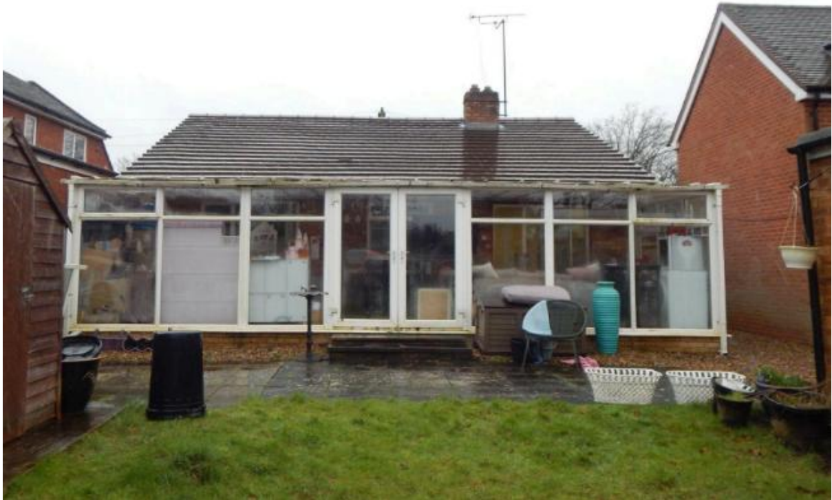
Image 3 – North facing elevation of the property
