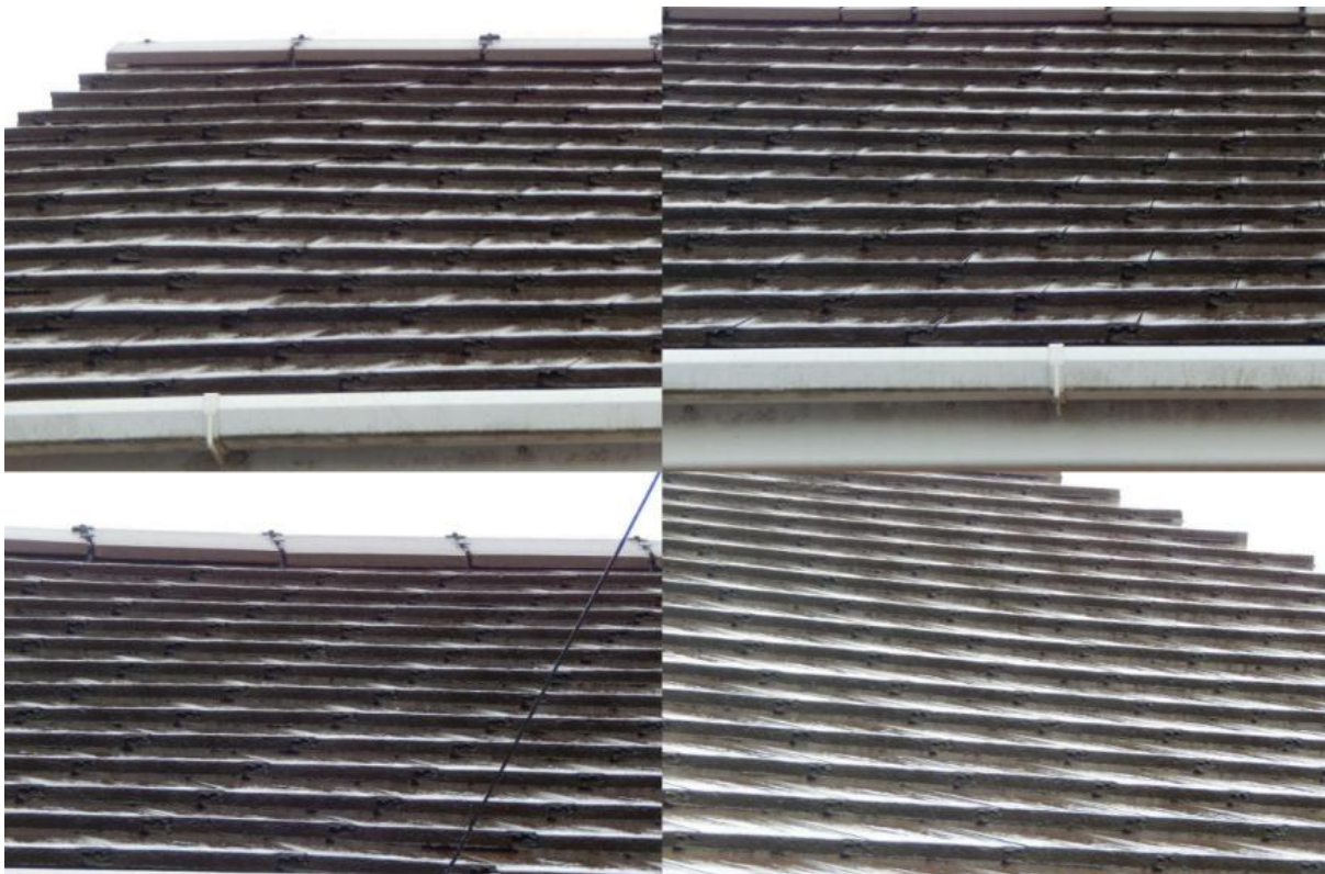
Image 2 – South facing roof coverings which have demonstrated no features of value to bats throughout
