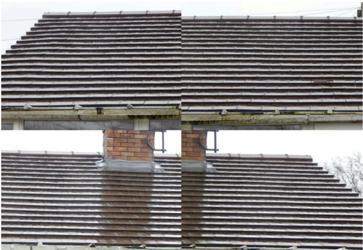
Image 4 – North facing roof coverings which have demonstrated no features of value to bats throughout
