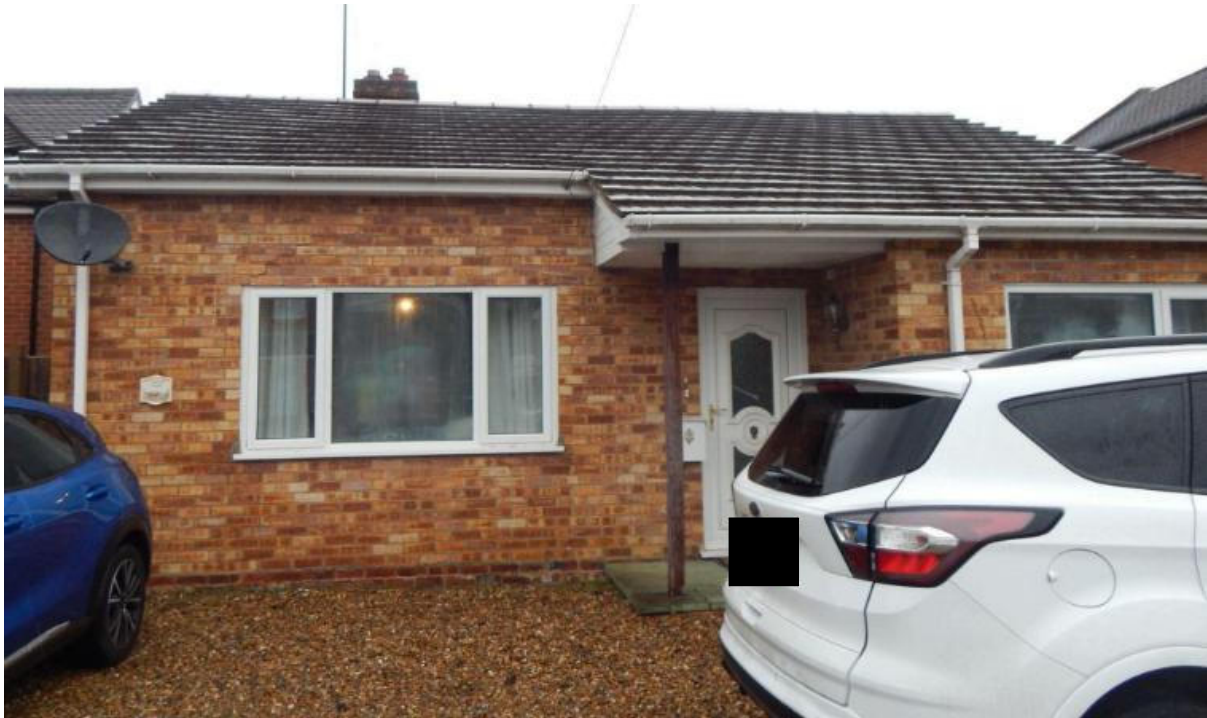
Image 1 – South facing elevation of the property
