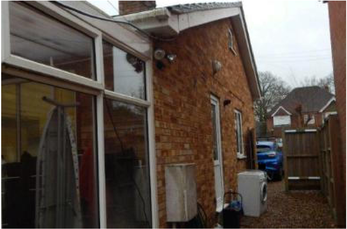
Image 7 – West facing elevation of the property
