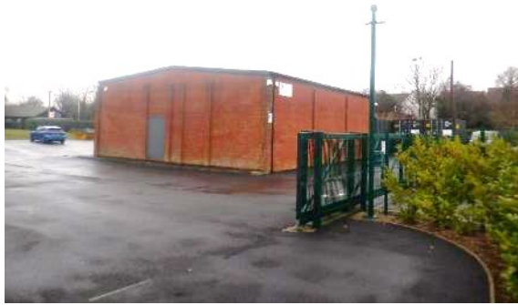
Photograph 4. Main commercial building used by LM Electrical Services on the south-western side of the site.
