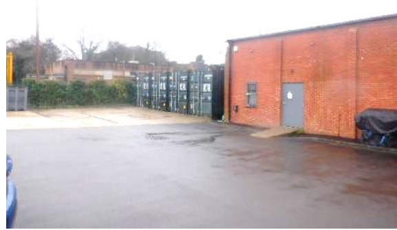
Photograph 5. Four storage containers to the south of the main building on concrete hardstanding and tarmac car parking facilities at the rear of the building.
