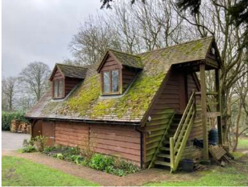
Photograph 3: Condition of roofing tiles of B3
