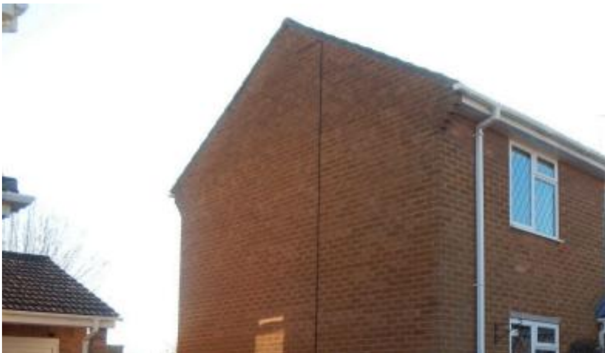
Image 6 – East facing elevation of the property
