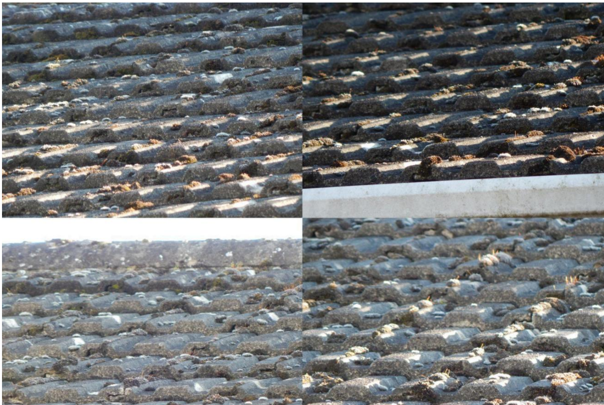
Image 2 – Views of the North facing roof coverings where no features of value to bats were observed
