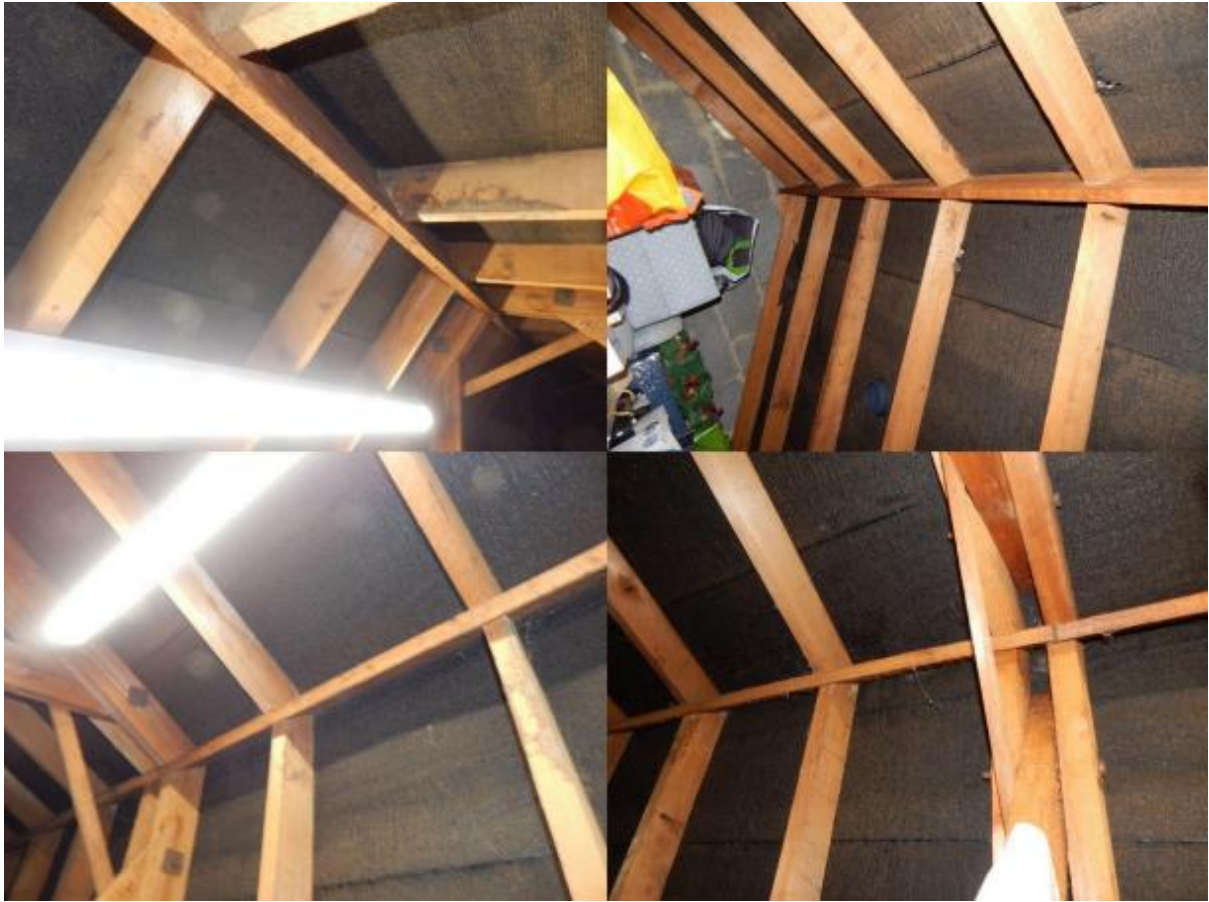
Image 9 – Internal view from within the main roof void spaces of the property
