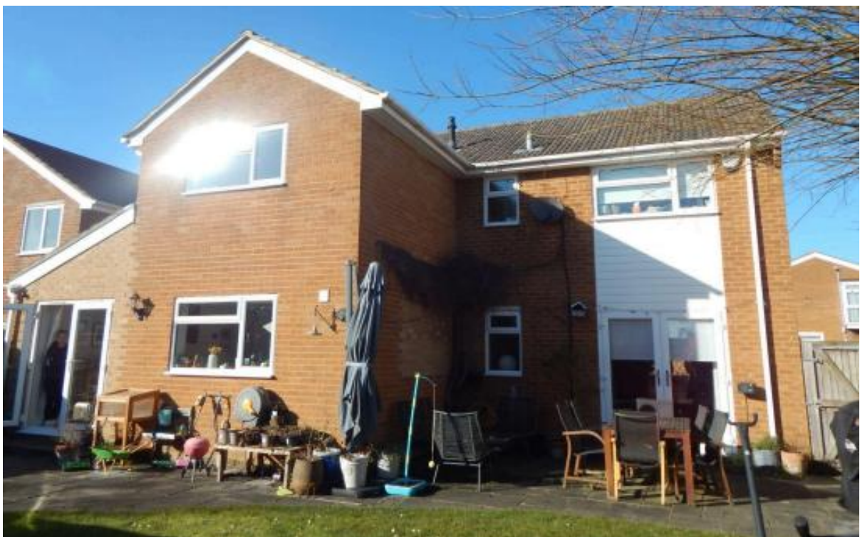
Image 4 – South facing elevation of the property
