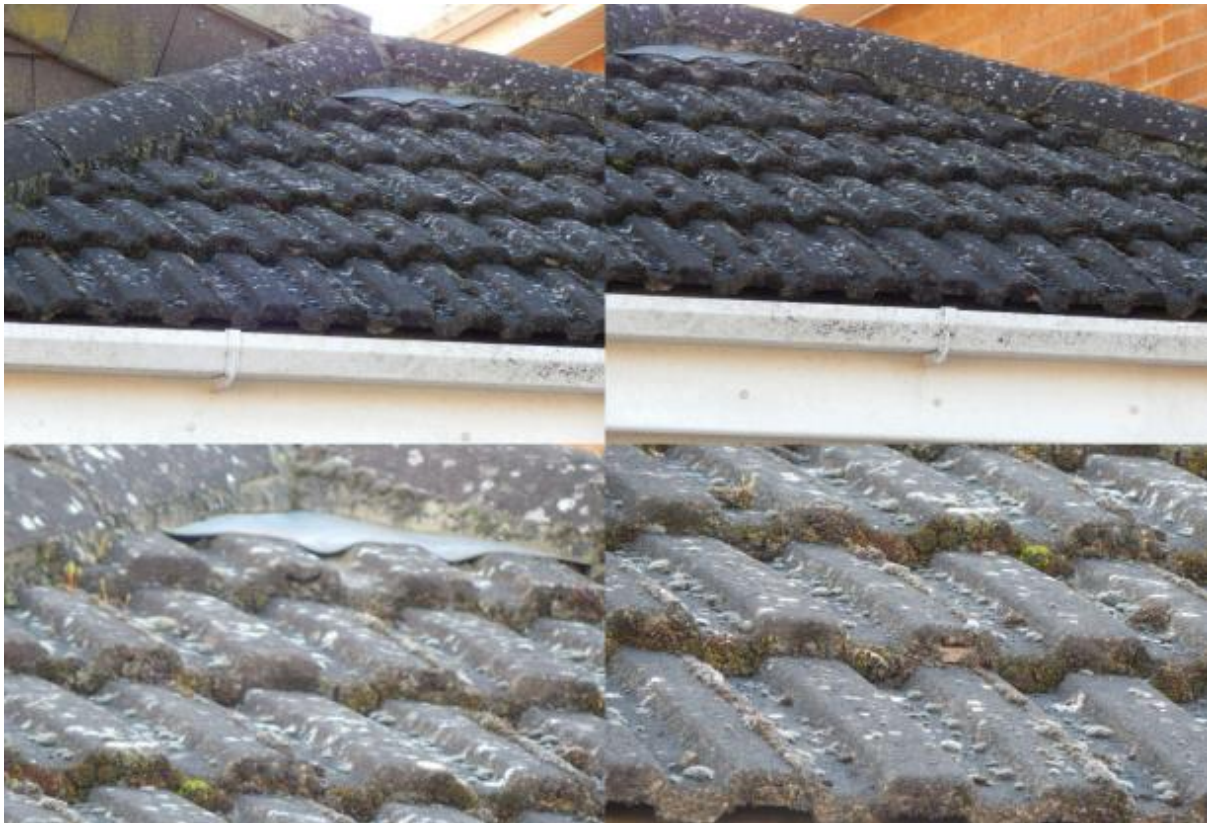
Image 3 – Views of lower North facing roof coverings where no features of value to bats was observed
