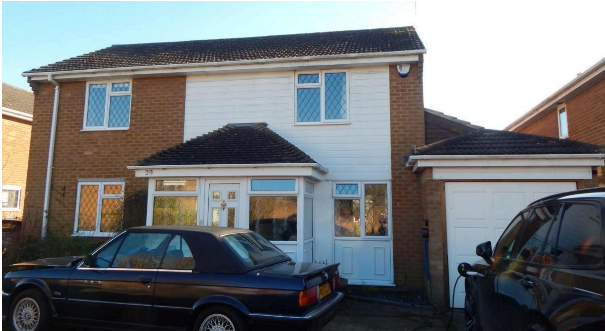
Image 1 – North facing elevation of the property
