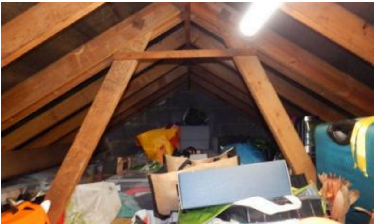
Image 10 – Internal view from within the main roof void spaces of the property
