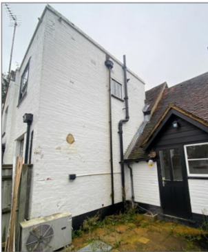
Image 25: West elevation of C20 extension
