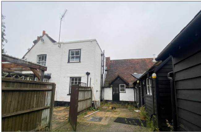
Image 22: North elevation of Barn and service yard
