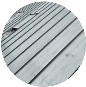
1. Standing seam metal roof
