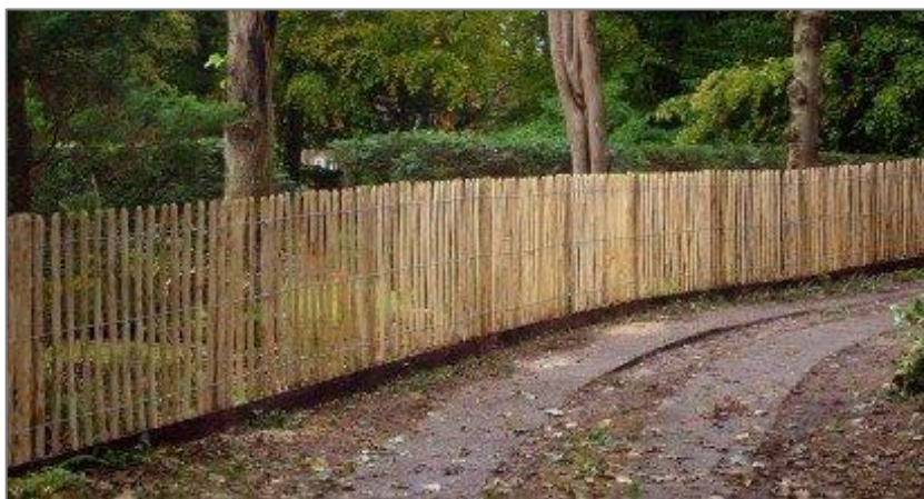
Figure 8, 3-wire ches-pale fencing
