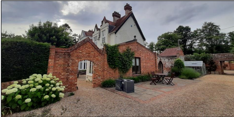
Photograph 2. The eastern elevation of Arborfield House. Also shown is the brick wall leading to the overhang (right side of image) and the southern and eastern aspect of the store, with a pitched roof.
