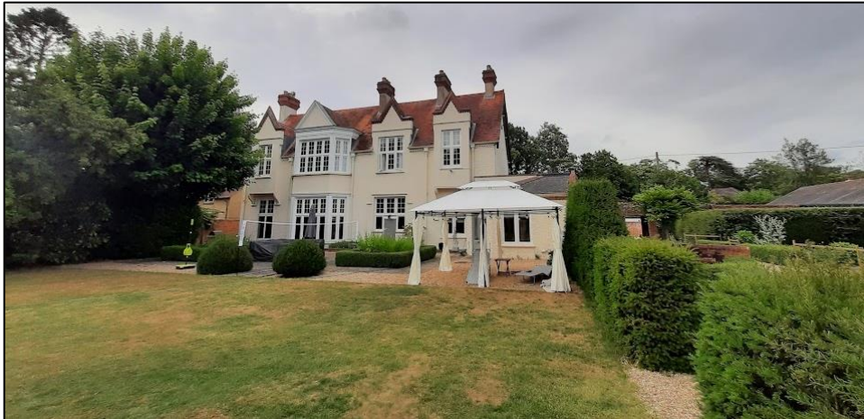
Photograph 1. The southern elevation of Arborfield House which is brick built and supports a hipped, gabled roof. Note the surrounding gravelled and hard-standing areas surrounding the property.
