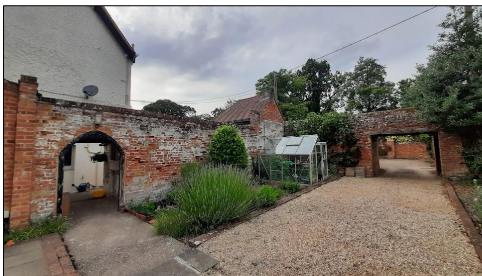
Photograph 8. The brick-built wall and southern aspect of the overhang.
