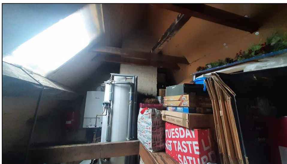
Photograph 6. Loft void one within Arborfield House.
