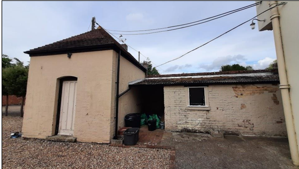
Photograph 13. The western and southern aspects of the store (left side of image) and the western aspect of the tool shed, with adjoining log store (centre and right side of image).
