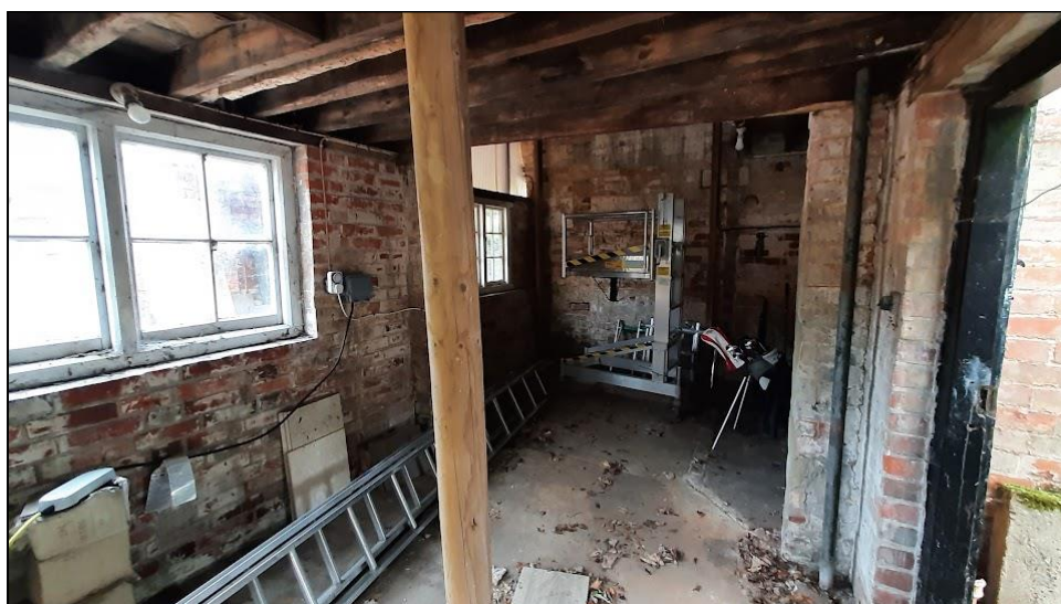
Photograph 21. The internal areas of the single garage/outhouse taken facing south.
