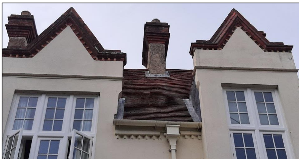
Photograph 5. An example of the gaps identified across the roof of the main house providing suitable bat access and roosting opportunities.
