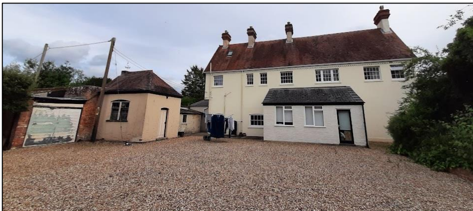
Photograph 3. The northern elevation of Arborfield House showing the single storey extension. Note the surrounding gravelled and hard-standing areas. Also shown are the north and western aspects of the store, with a pitched roof, hipped roof and the single garage/outhouse (to the left of the image).
