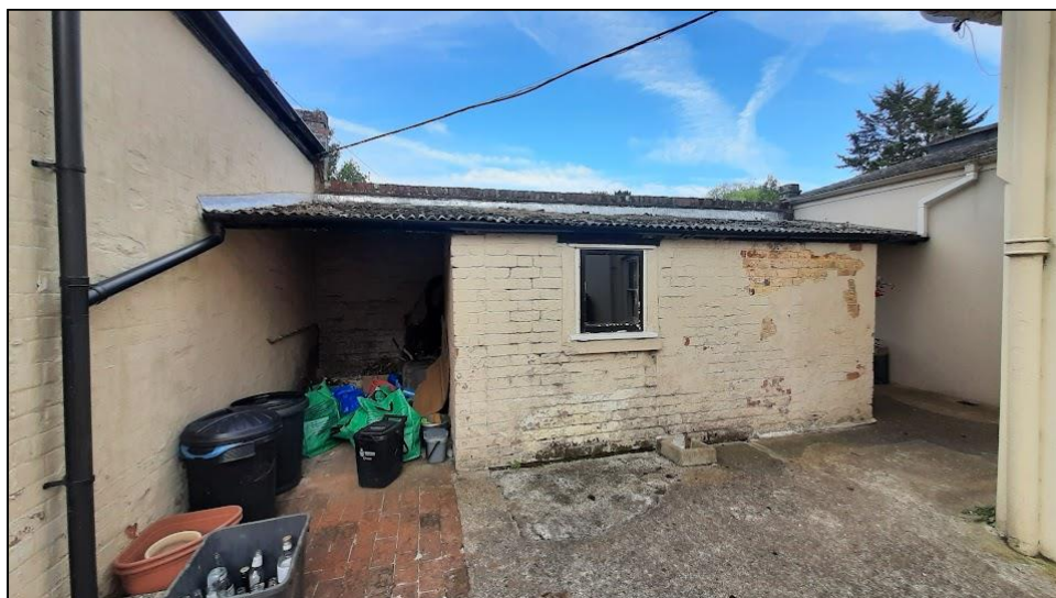
Photograph 22. The western aspect of the tool shed, with adjoining log store.
