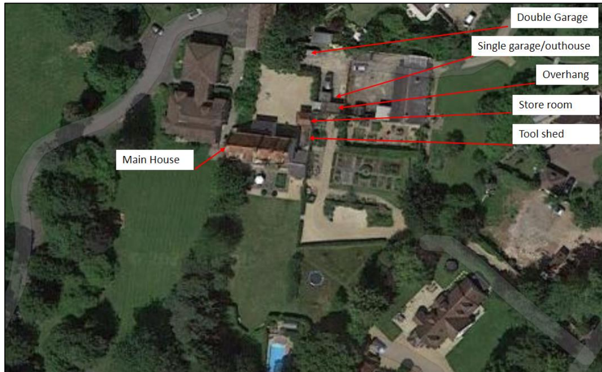
Figure 1. Aerial image of Arborfield House, Reading, with the surveyed buildings labelled for the purposes of this report.
