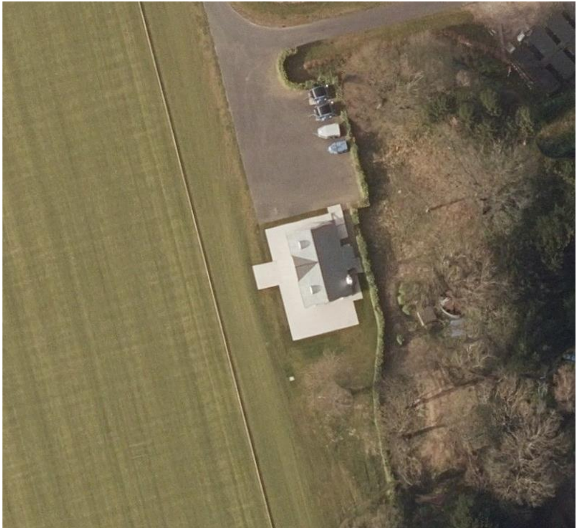
Fig 17 – Date verified aerial photo from Getmapping.co.uk (dated 05/04/2020) showing the pavilion, terrace and paved hard area complete
