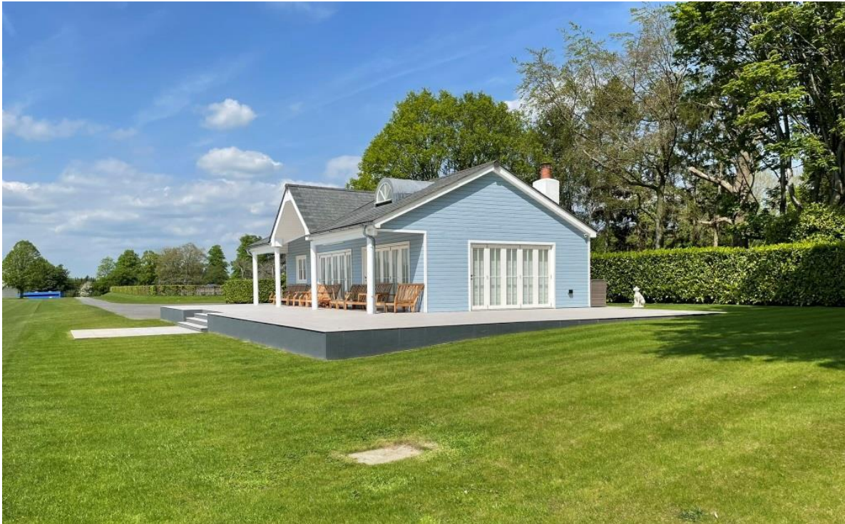
Fig. 2 – Pavilion building (May 2024) – South west elevation
