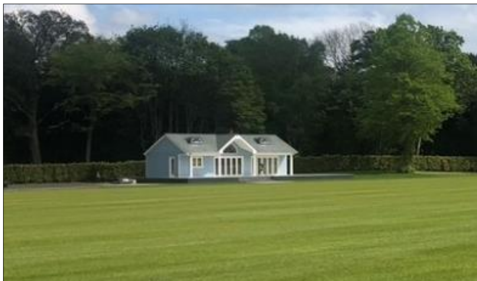
Fig 15. – Enlargement of photo taken by [REDACTED] (Polo Manager) on 3 May 2019, showing the completed pavilion building, raised terrace and (ground level) hard paved area in front
