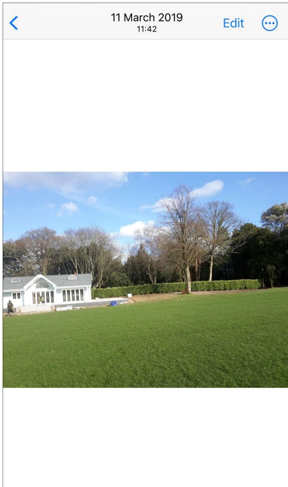
Photo. 2 – Shows pavilion completed, with some works still on-going in and around the terrace and ground level paved area (to the front)
