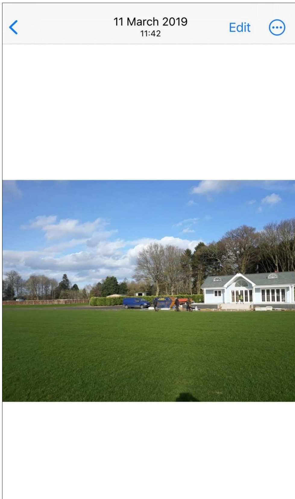
Photo. 1 – Shows pavilion completed, with some works still on-going in and around the terrace and ground level paved area (to the front)
