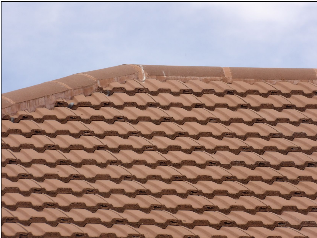
Figure 4. Example of interlocking roof and sealed ridge/hip tiles. 33 Stanton Close, Earley. 16.07.25
