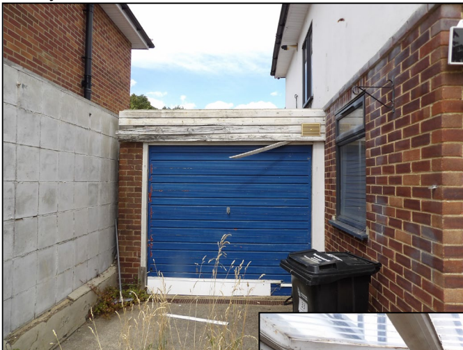
Figure 10. Garage and internally view of corrugated Perspex roof. 33 Stanton Close, Earley. 16.07.25
