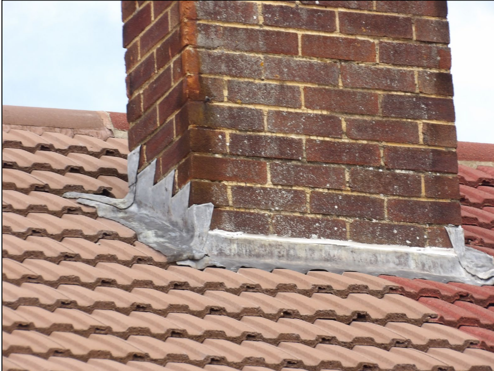
Figure 5. Example of sealed lead flashing. 33 Stanton Close, Earley. 16.07.25
