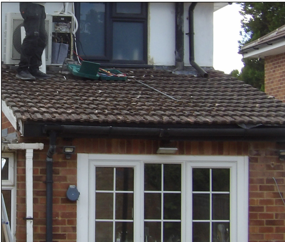
Figure 8. Roof of rear, mono-pitched extension. 33 Stanton Close, Earley. 16.07.25
