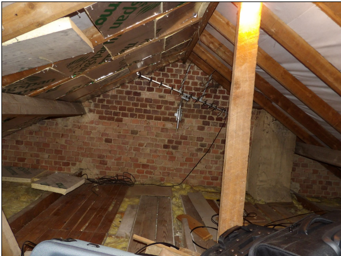
Figure 11. Example of loft space and insulation/membrane lining. 33 Stanton Close, Earley. 16.07.25
