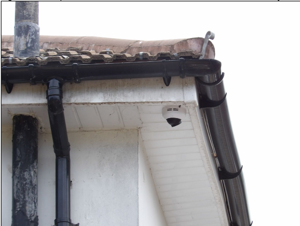
Figure 6. Example sealed uPVC soffits/fascias. 33 Stanton Close, Earley. 16.07.25
