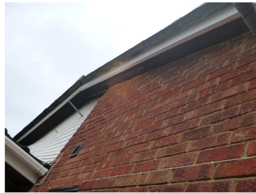
Photograph 8. Sealed soffits throughout (northeastern elevation)
