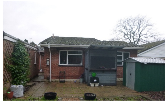
Photograph 2. Rear elevation, viewed from the southeast.
