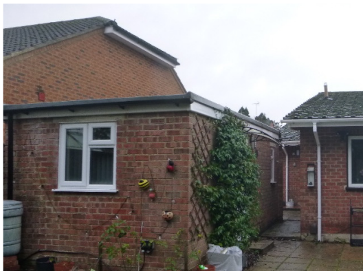
Photograph 9. Flat roof garage.
