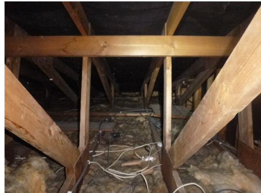
Photograph 12. Roof lined with fibreglass
