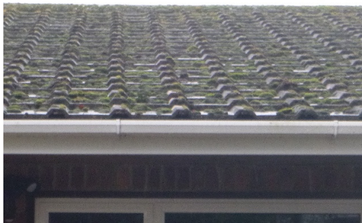
Photograph 3. Tight fitting interlocking concrete tiles (rear southeast elevation)
