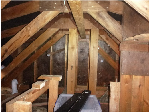
Photograph 10. Trussed roof construction
