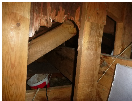
Photograph 14. Inaccessible space behind the southwestern gable.
