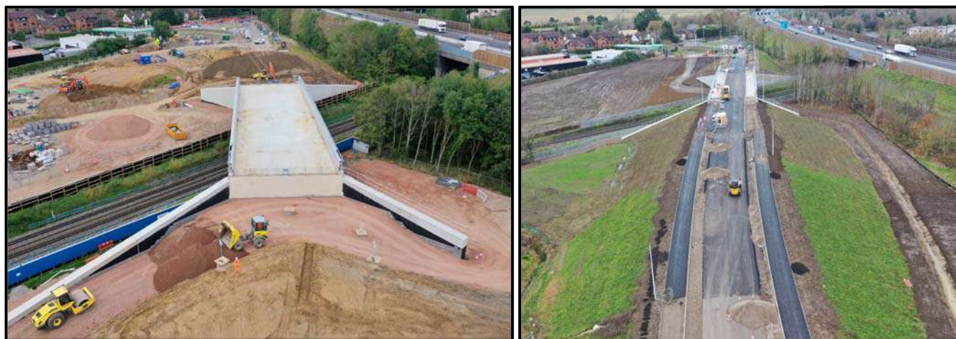
Figure 32: Typical example backfill to the bridge and final groundworks and surfacing to the bridge
