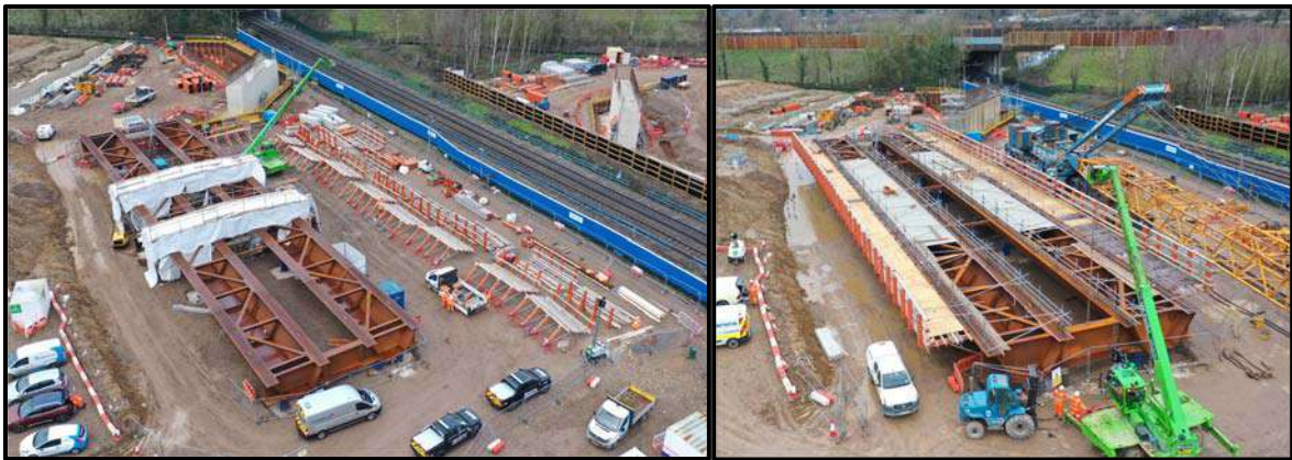
Figure 28: Typical example welding of the beams and setting up the cantilever formwork for installation to beams
